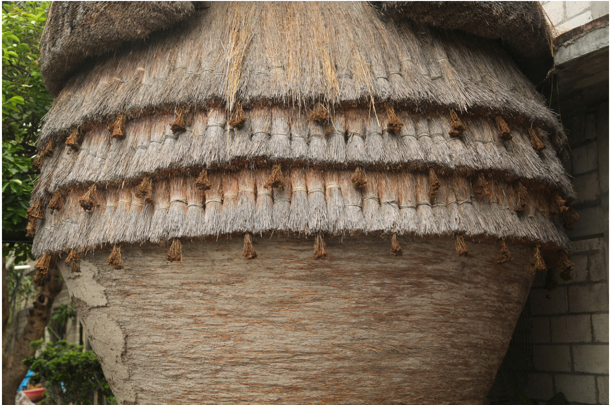
Figure 7. Layer of dry zacate that prevents animals from climbing and entering the cuexcomate . Photograph Project Crafts of Pre-Hispanic Mexico. Ethnoarchaeological Study Final Stage.
