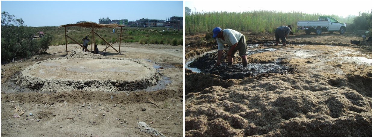
Figure 6. Raw materials collected in the circle (left) and mud mixing/kneading (right) (M. Lorenzon).
