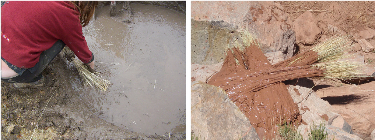
Figure 9. Opening of the straw to be dipped in the mud (a), and the arrangement of the guayas before being lifted onto the roof (b).
