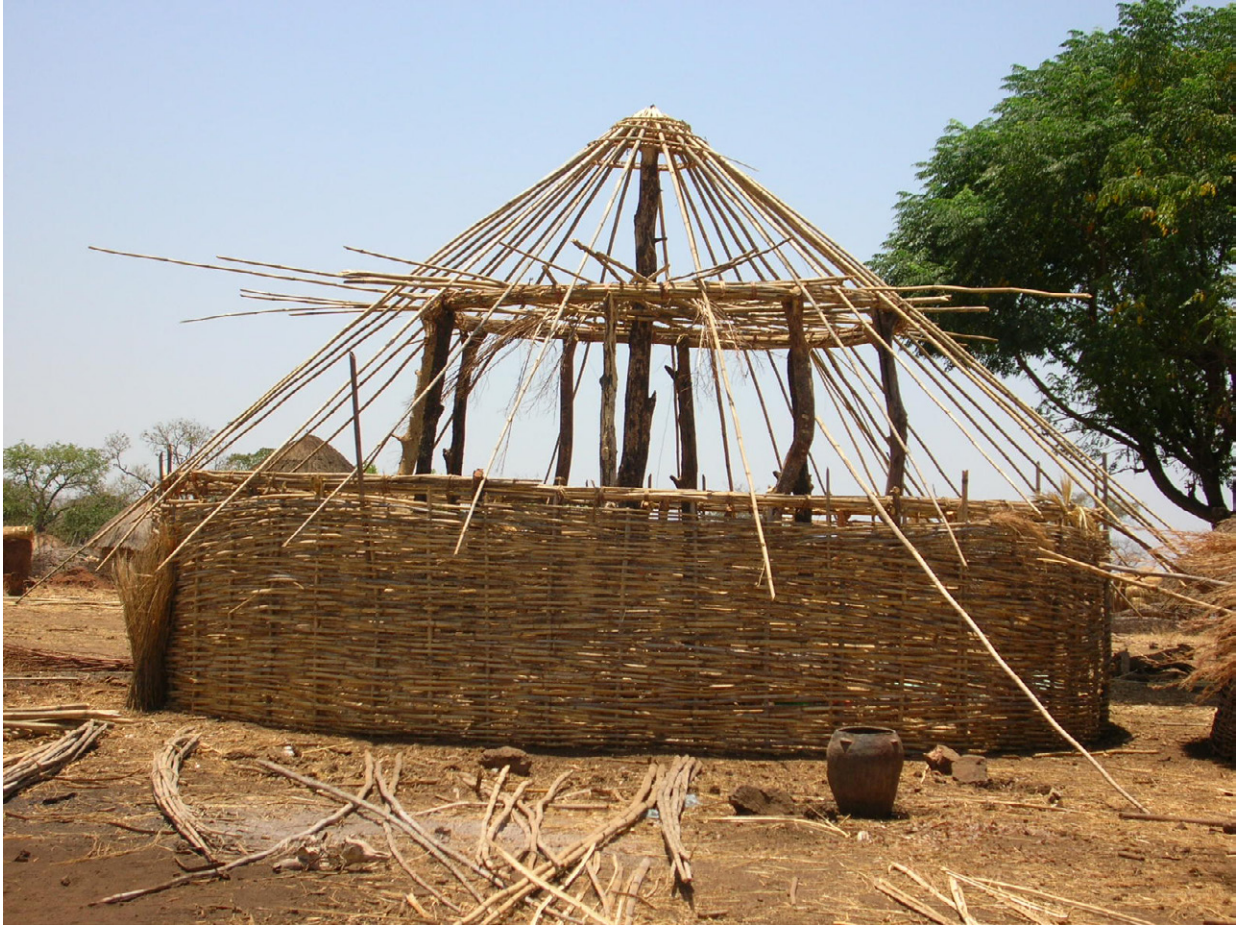
Figure 6. Gumuz hut under construction, showing the concentric structure of posts supporting the roof from the inside. Photograph by Xurxo Ayán Vila.
