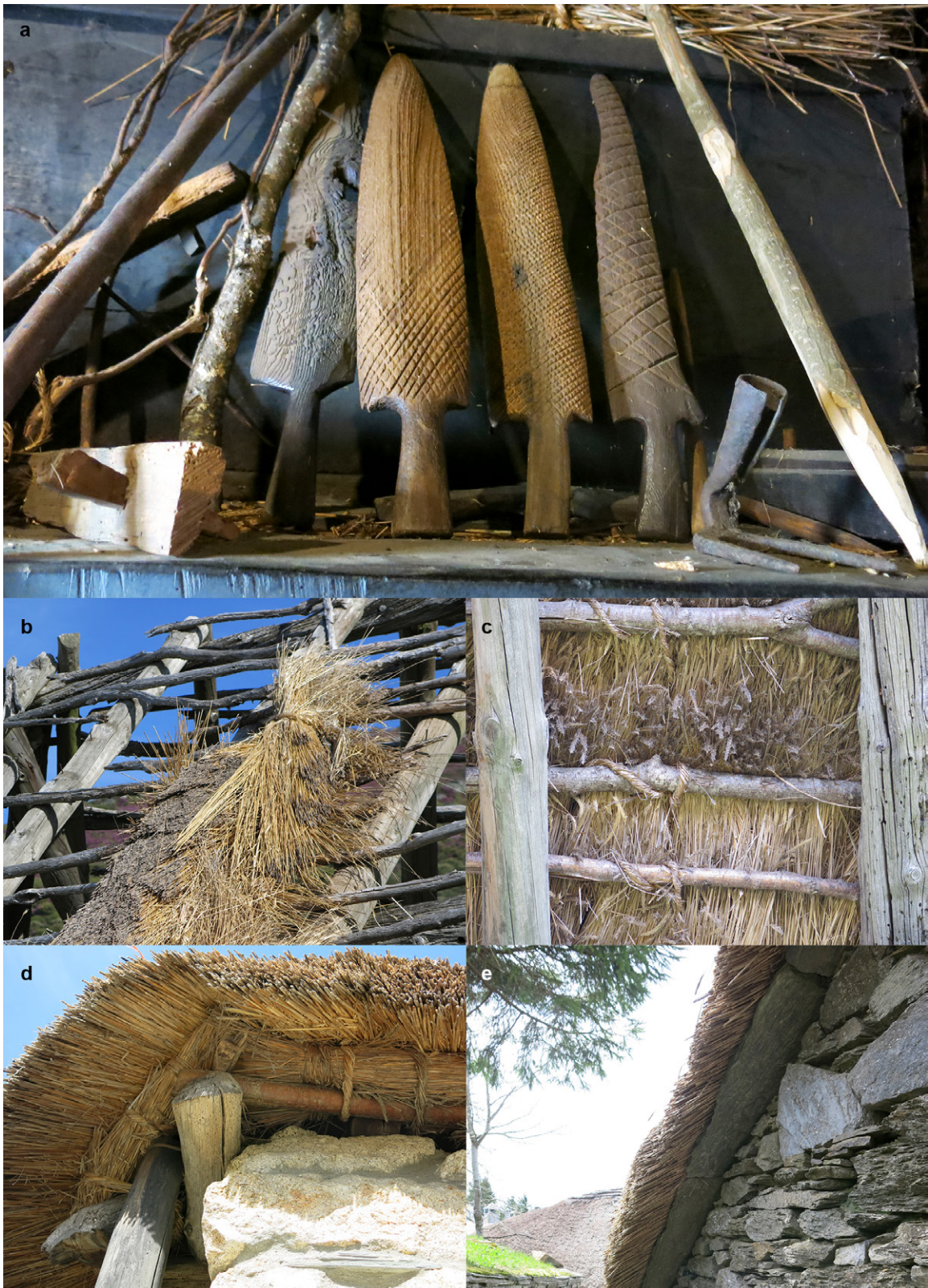
Figure 9. Thatching a palloza : a) wooden leggets from Piornedo (Lugo); b) partially collapsed palloza in Campo d'Agua (León), with the thatch held in place by straw ropes; c) thatch secured with straw ropes in Campo d'Agua (León); d) straw cord used to lift the thatch in Campo d'Agua (León), and e) stone slabs used to lift the thatch in O Cebreiro (Lugo).
