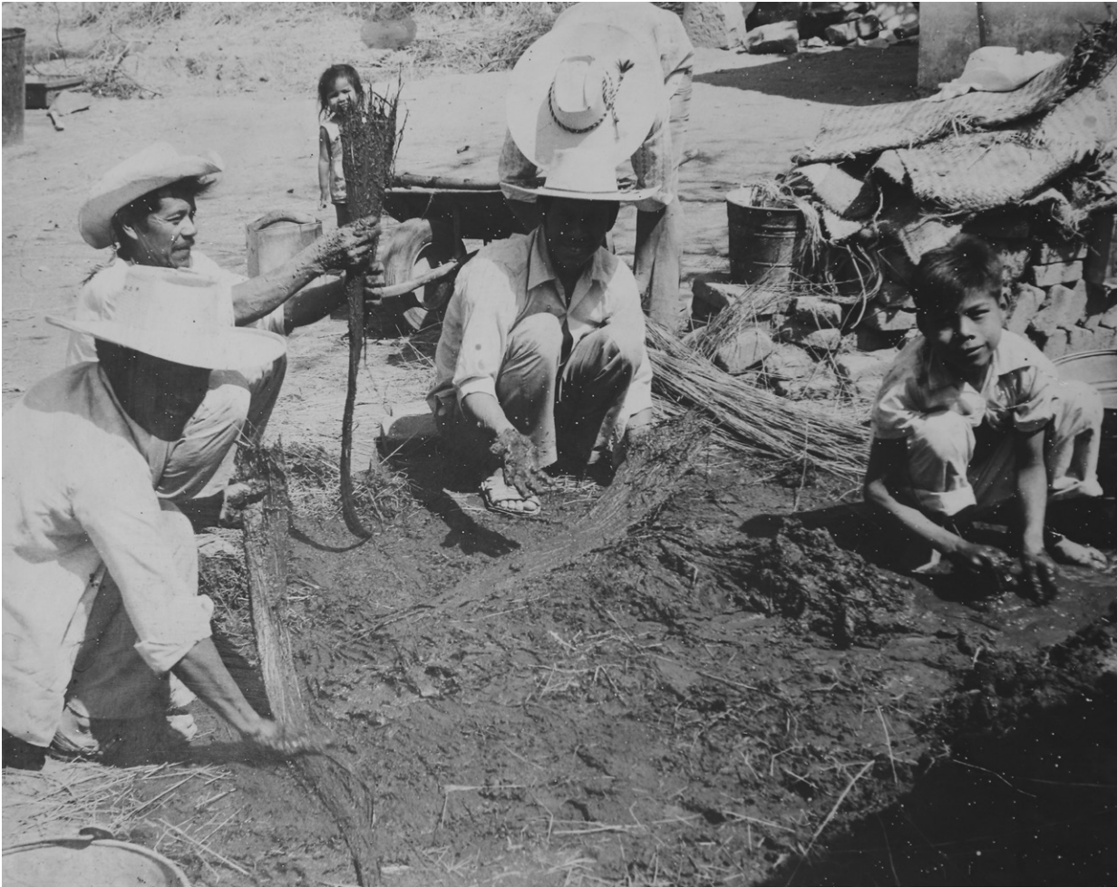
Figure 6. Preparation of zacate ties for the construction of a cuexcomate body. Photograph located at the municipal agency of the town of Chalcatzingo, Morelos. Photograph archive Crafts Project of Pre-Hispanic Mexico. Ethnoarchaeological Study Phase 2.
