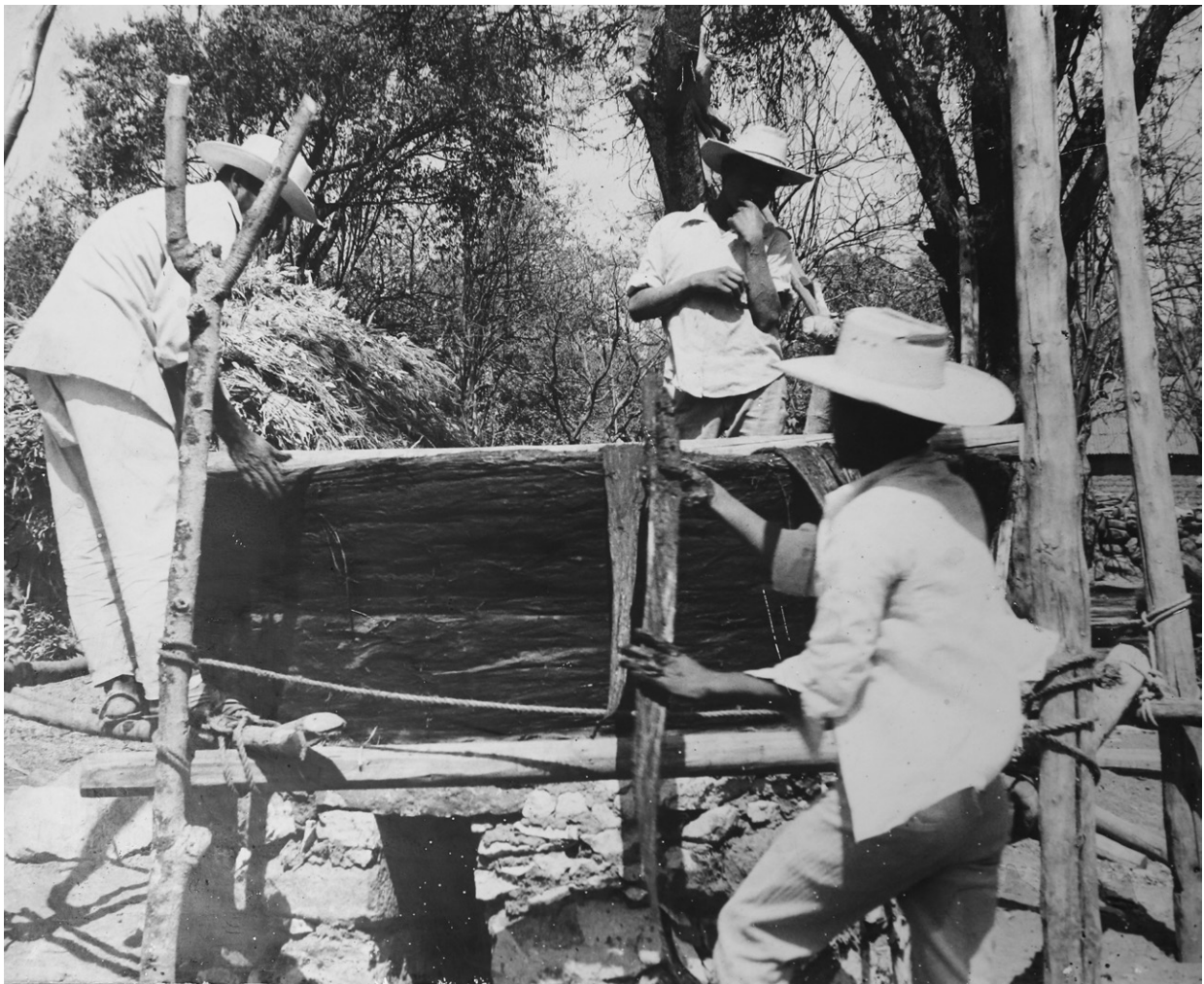
Figure 5. Scaffold constructed around a cuexcomate . Photograph located at the municipal agency of the town of Chalcatzingo, Morelos. Photograph Project Crafts of Pre-Hispanic Mexico. Ethnoarchaeological Study Final Stage.
