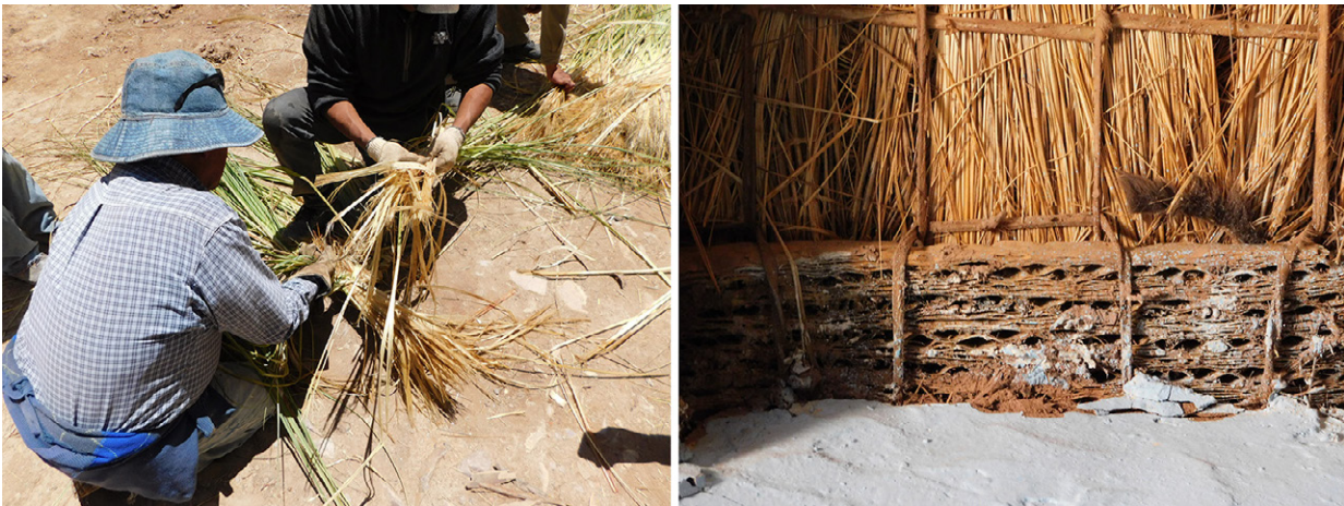
Figure 6. The weaving process of the cortadera in a historic house in Yavi (a), and the weaving process of the tientos mesh that supports the layer of straw in the Church of Tabladitas (b).
