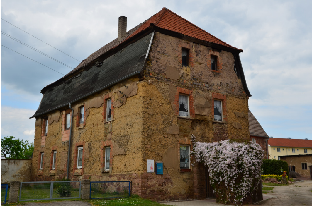
Figure 2. Lettewitz, Saalekreis district, Saxony-Anhalt, a typical late baroque manor house (c. second half of the 18th century). A load-bearing cob wall rises above a stone base (porphyry) to form two full storeys. As gables are difficult to construct using the cob technique, other earthen building techniques or materials (in this case, stone masonry) were generally used. (© GOLEHM, LDA Saxony-Anhalt, F. Knoll).
