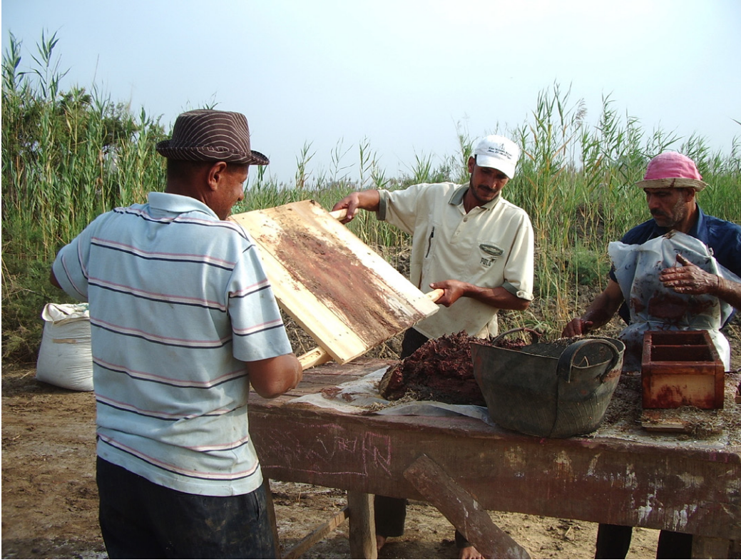
Figure 7. Transportation of the mud mixture (M. Lorenzon).
