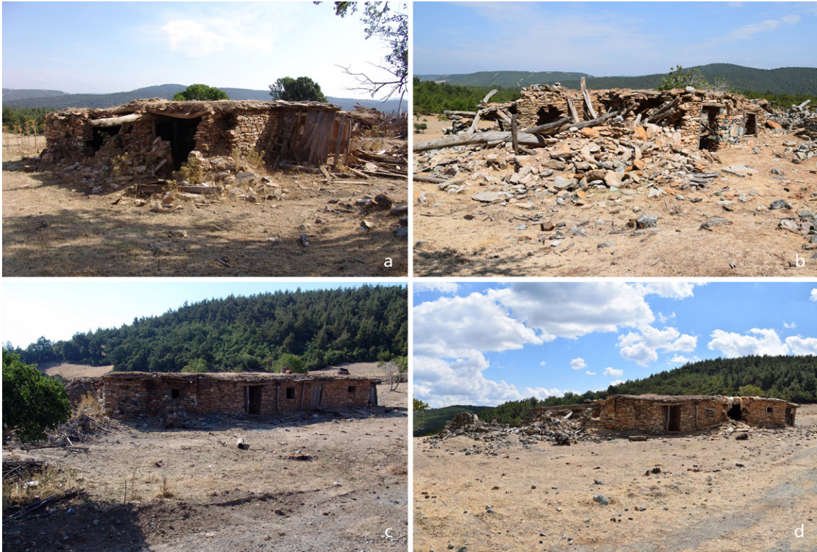
Figure 14. (a) Condition of building 1C on 8 August 2006 and (b) on 19 August 2016; (c) southern building complex of Armutalan from a northwestern perspective on 8 August 2006 and (d) on 26 August 2016.
