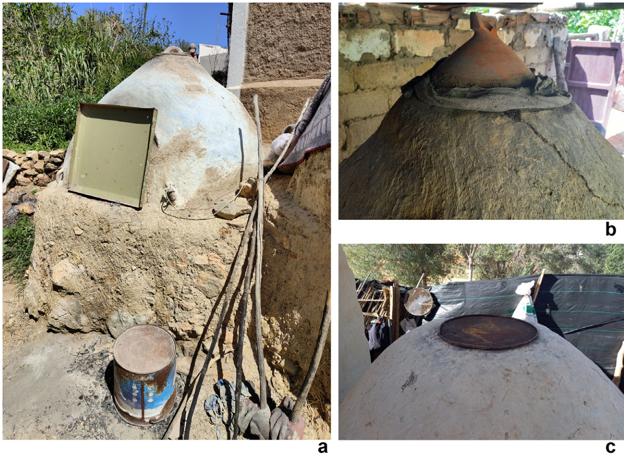
Figure 7. Examples of covering systems for the oven openings. a) View of Oven 7, which possesses two side handles and a ceramic (up) and a square metallic (down) removable lid. b) Ceramic lid of Oven 6 made by reusing a tajine. c) Metallic lid of Oven 3 with a rounded shape.
