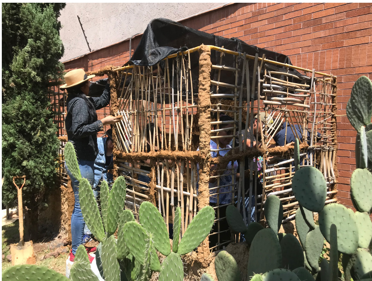
Figure 3. Building the orchid house with the wattle and daub technique.
