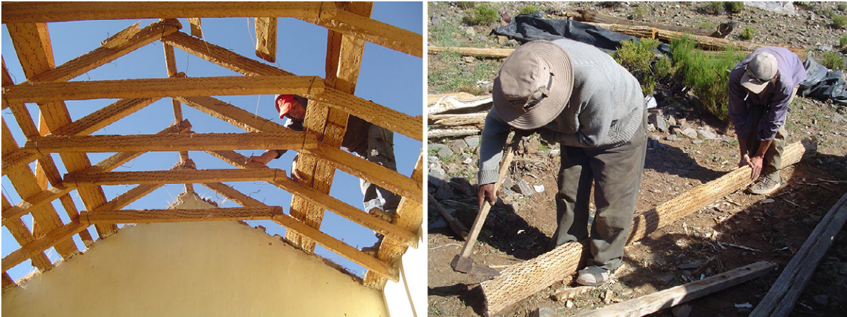
Figure 4. Assembling a structure with cardón boards (a) and processing the wood (b), both in Susques.
