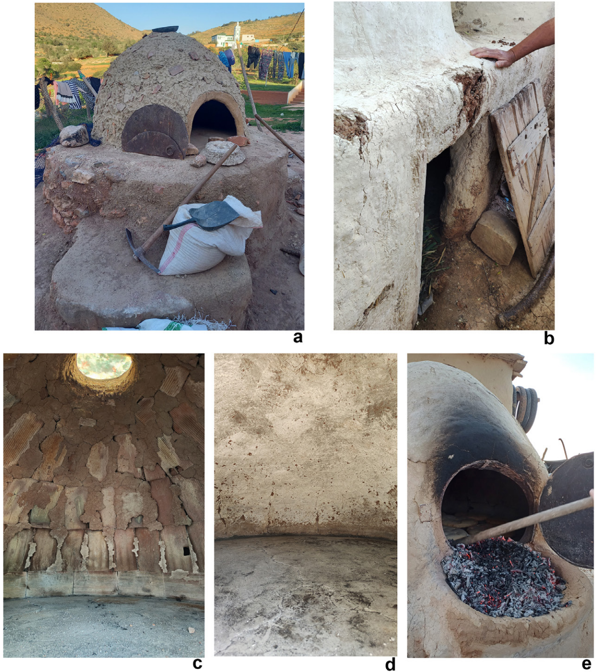
Figure 6. Details of the different parts of the ovens. a) Oven 9, whose dome still lacked the external earthen layer. b) The podium of Oven 3, which is hollow and is used as a rabbit hutch. c) Interior view of the dome of Oven 3, whose inside is built entirely of bricks. d) Interior view of the dome of Oven 7, whose inside is built entirely of earth. Its combustion surface is made of clay without straw. e) View of the ledge of Oven 3 while in use.
