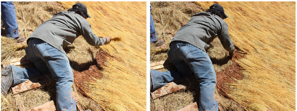
Figure 11. Succession of movements for the placement of the guayas on the roof.
