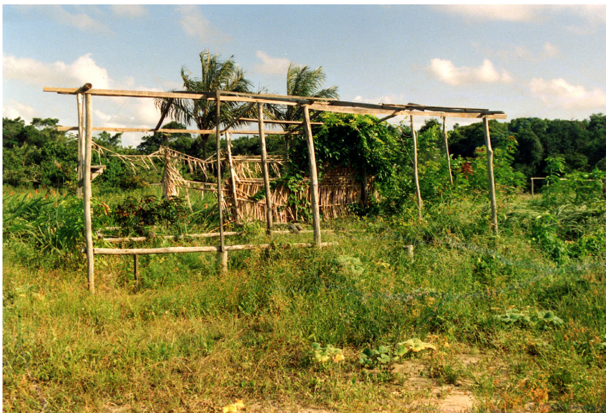
Figure 10. House ruins in Savane Maillard (photographs by S. Rostain).
