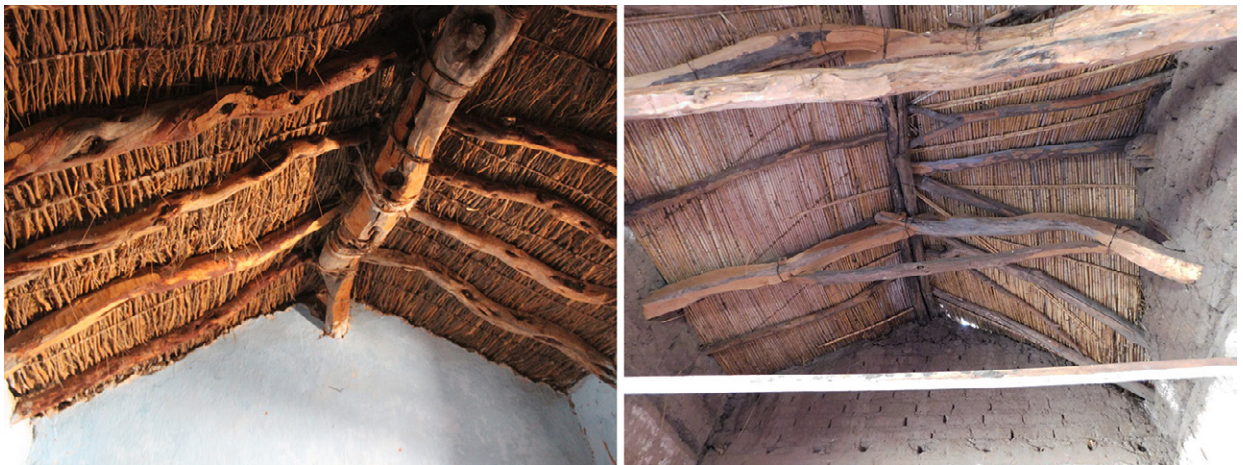
Figure 3. Structure made of queñoa wood with rods on top in Tabladitas (a) and its combination with other species in Yanallpa (b).
