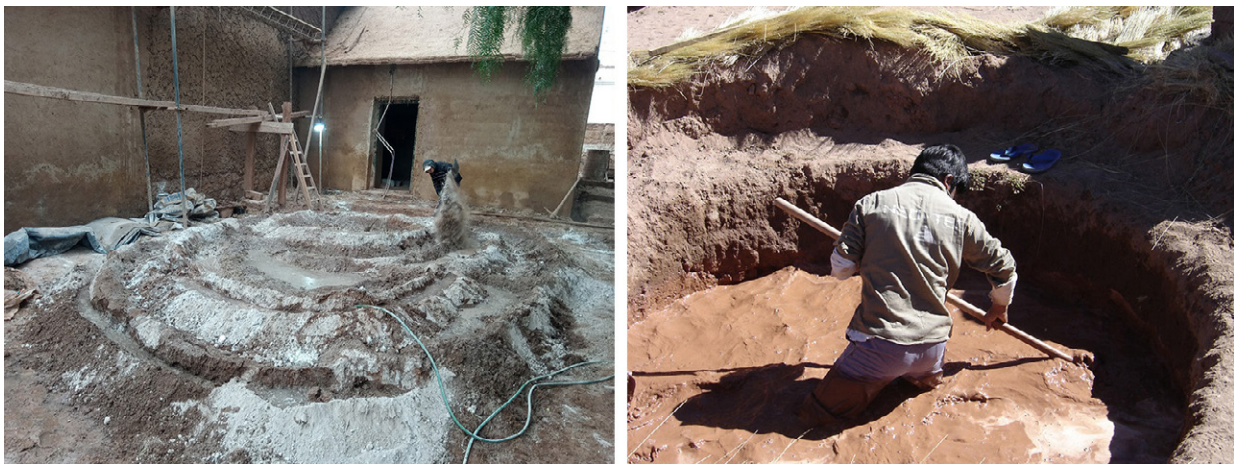
Figure 8. Preparation of the mud for the torta de barro , with the addition of water, in Uquía (a) and the pit with viscous material for the guayado of a house in Susques (b).
