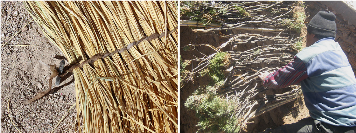
Figure 5. Weaving with straw in Conchi Viejo (a) and with tola branches in Rinconada, tied with leather strings (b).
