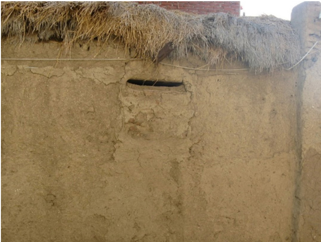
Figure 4. A former window has been blocked to allow less sun in and control ventilation (Buto, Lower Egypt). Photograph by the author.
