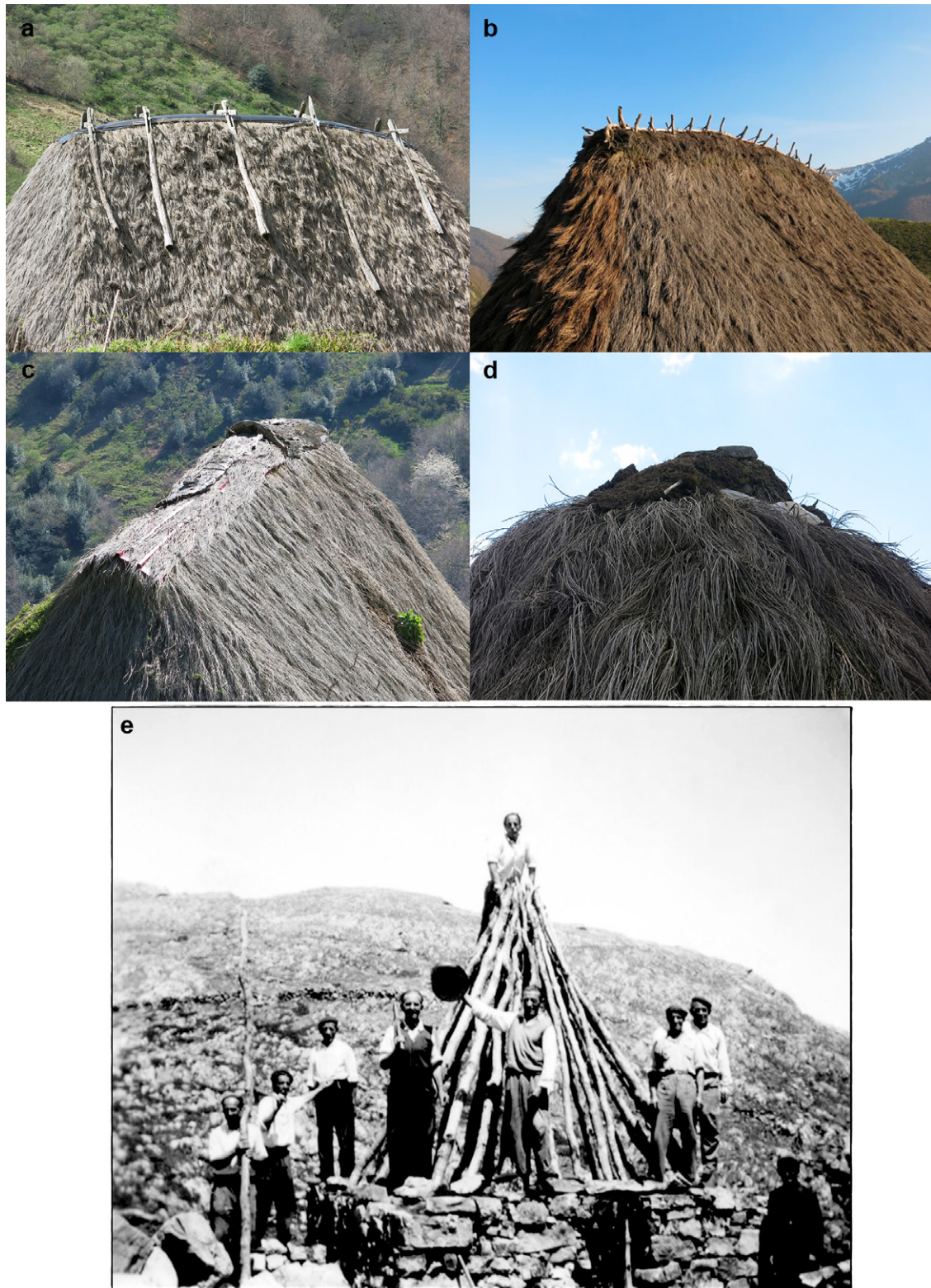
Figure 6. Social implications of broom thatching. 1) Different ways to secure a broom thatch: a) planks and logs ( zancas and xugos ) in La Pornacal (Somiedo, Asturias), b) logs and sticks ( llatas and gabitos ) in Murias Llongas (Somiedo, Asturias), c) dry logs ( tuerus ) in Tuiza (Teverga, Asturias) and d) turf ( tapines ) in Sousas (Somiedo, Asturias); 2) Collaborative structure rebuilding: chozo in Peñalavera (Acevedo, León, courtesy of Ángel Cimadevilla).
