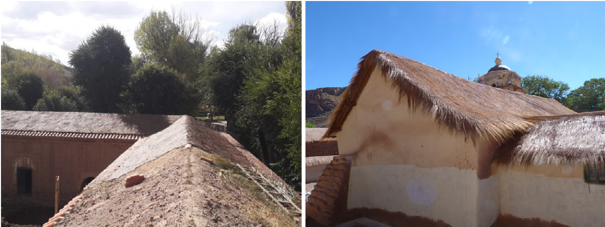
Figure 2. Views of the torta de barro roof at the Casa del Marqués in Yavi (a) and the guayado at the Church of Susques (b).
