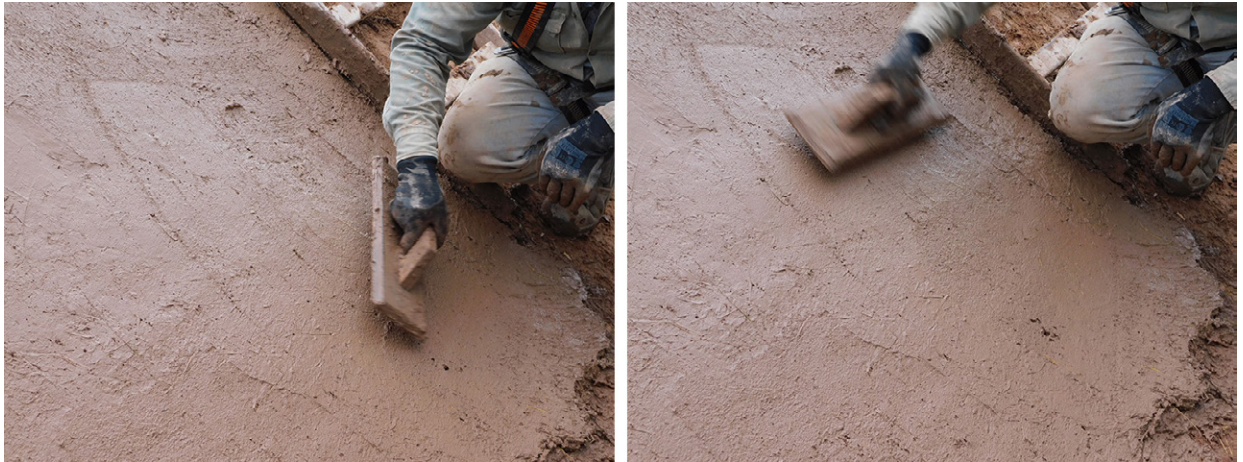
Figure 10. The technical gestures for the smoothing of the mud in the torta de barro process of the Church of Uquía.
