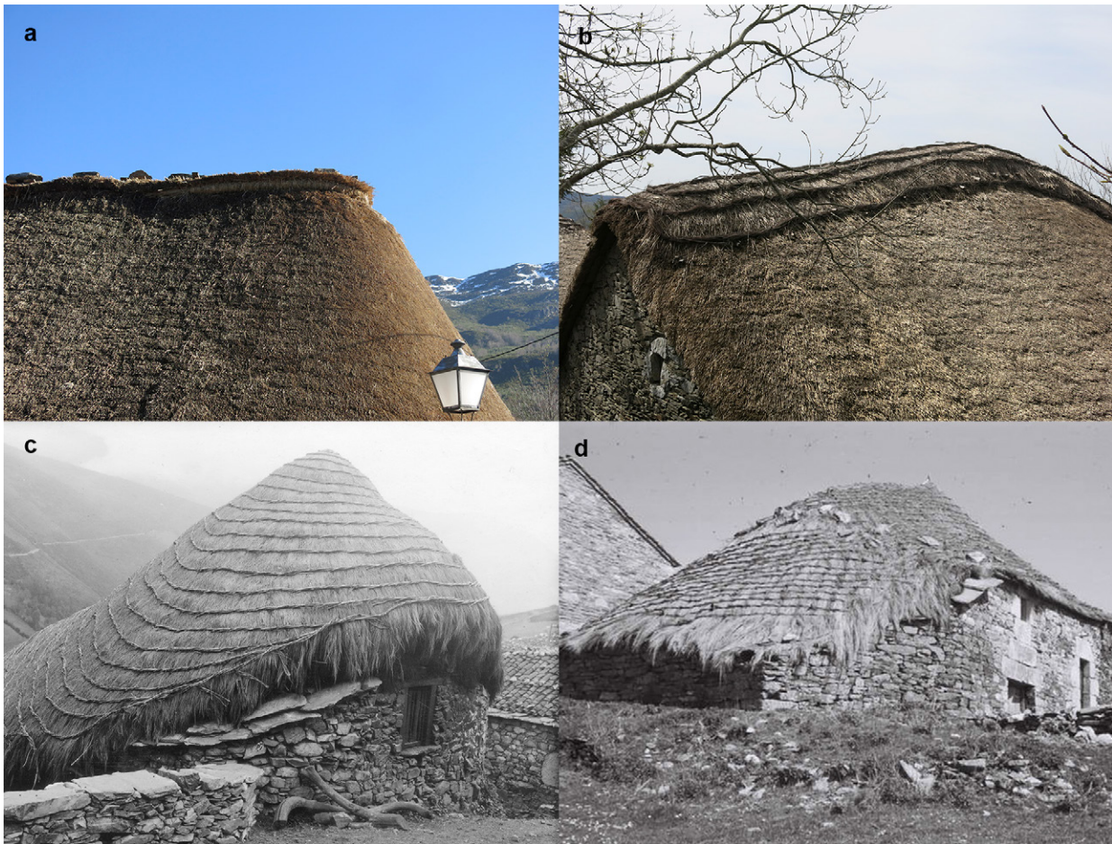
Figure 10. Methods for securing a rye straw thatch. Teitado a paleta : a) straw cord fixed with ropes and stakes (Balouta, León) and b) interwoven branches tied at the top (O Cebreiro, Lugo). Teitado a baguna : c) interwoven branches tied across the entire thatch (Genestoso, Asturias, photograph by Fitz Krüger, 1927, courtesy of Museo del Pueblo de Asturias) and d) mesh of interwoven branches and straw ropes secured with rocks (O Cebreiro, Lugo, photograph by Manuel Chamoso Lamas, courtesy of Real Academia Gallega de Bellas Artes).
