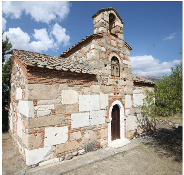
Fig. 14. Panagitsa church built with architectural blocks and steles from the Artemision (A. Voegelin, ESAG).
