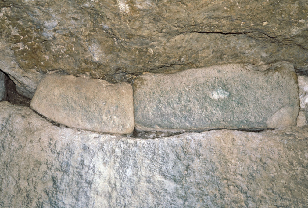
Figure 7. View of two stones inserted between the top of the chamber wall and the base of the capstone in the Bounias hypogeum Image: X. Margarit 2016.
