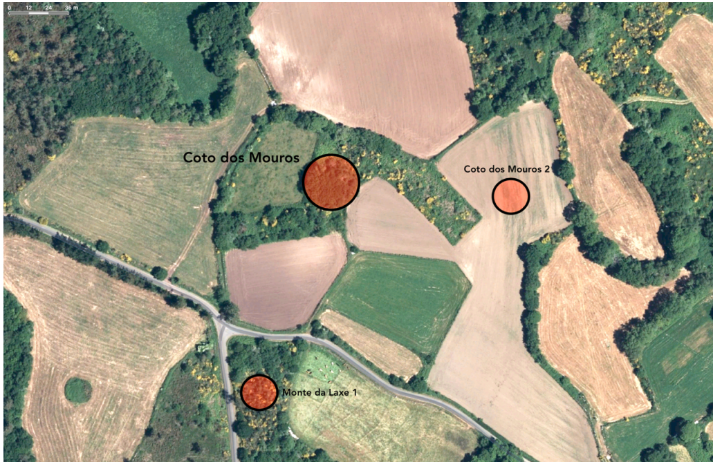
Plate 9. Aerial photograph of the Coto dos Mouros monument (BIC). Note the agricultural works throughout the area, which seriously affect another listed site (Coto dos Mouros 2). All three sites are included in a "protection area" recognised by the legislation for listed sites (or BIC).
