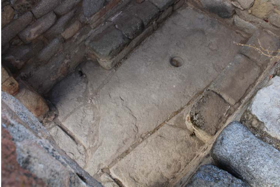
Figure 2 – San Pedro de La Mata, Toledo. Interior view of the apse from the south. The marks of the first row of chancel screens and the circular support of the altar are visible on the granite floor. The benches attached to the north and south walls were probably added in a later construction phase (P. Díaz Gutiérrez).
