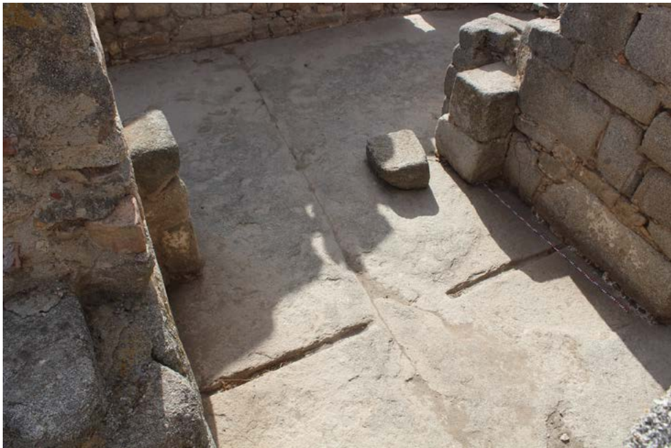
Figure 3 – San Pedro de la Mata, Toledo. Second row of chancel screens marks, viewed from the southeast. These separated the choir from the rest of the nave (P. Díaz Gutiérrez).
