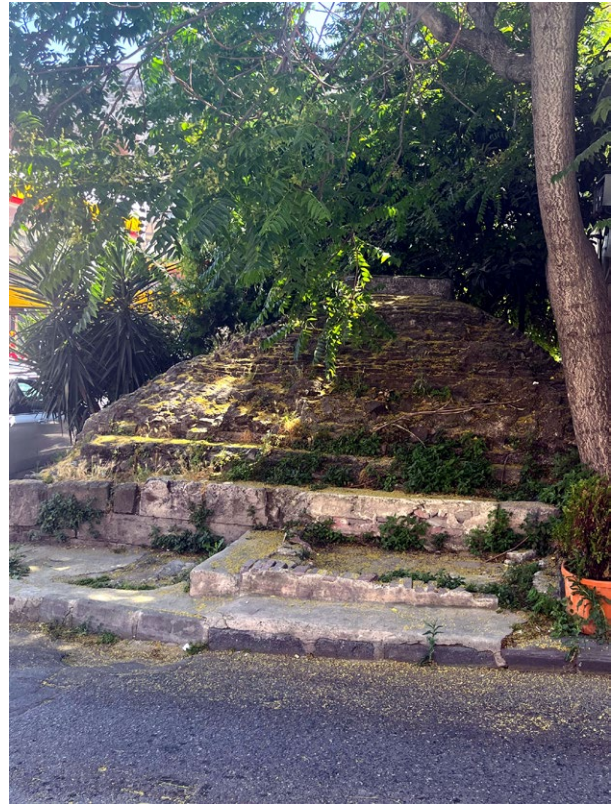
Figure 9. Dome of the Tezgâhçılar taksimi (Tezgâhçılar distribution chamber), 15th century, near the Valens Aqueduct, situation in 2024 (Photo. Mariëtte Verhoeven).
