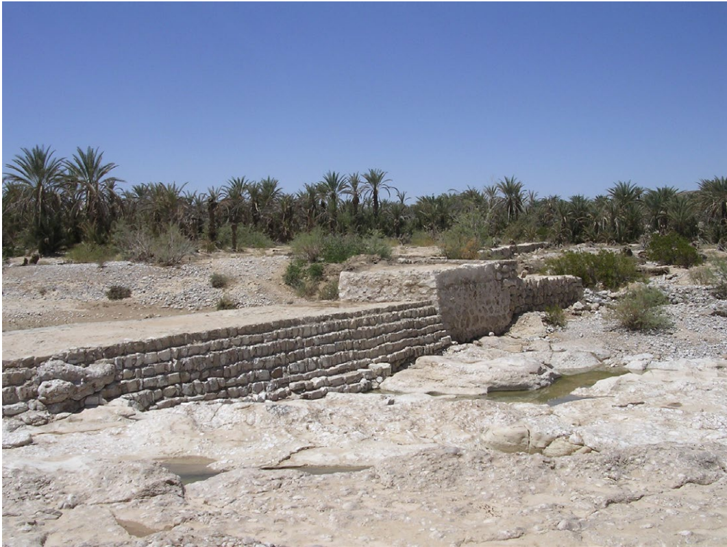
Figure 5. Dam slowing water from sayl flashfloods in Ghayl Bin Yumain, Hadramawt, Yemen (photo. M. Harrower, 2005).
