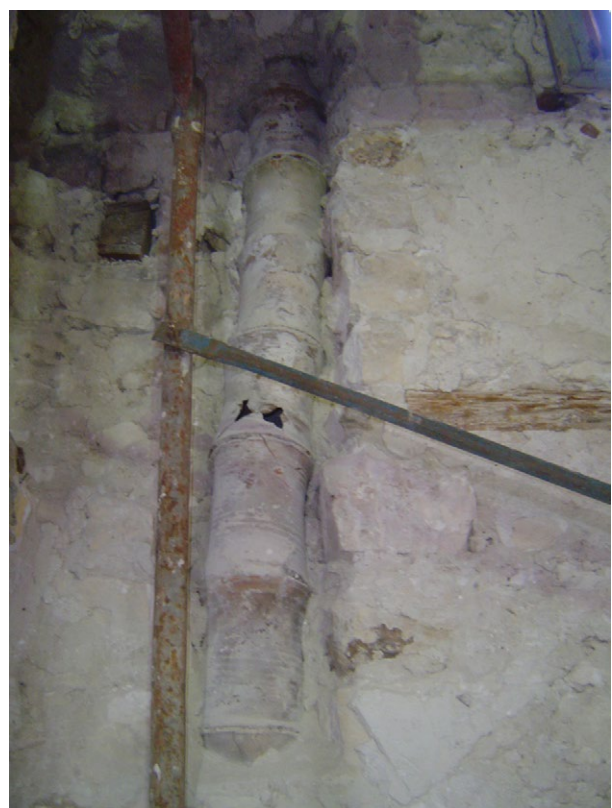
Figure 10. Rainfall harvesting technique associating with a cistern under Hajj Terbana Mosque (1097AH/1685CE).
