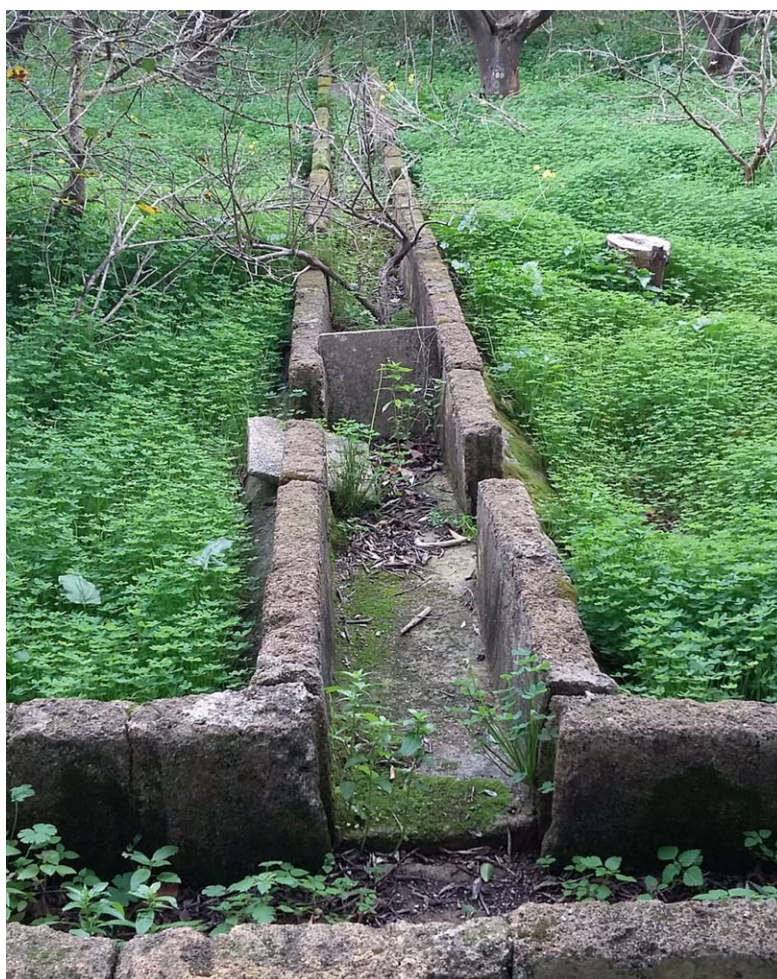
Figure 4. Sicilian traditional irrigation systems: an abandoned saja (water channels) inside the Favorita Park in Palermo (photo. A. Castrorao Barba).
