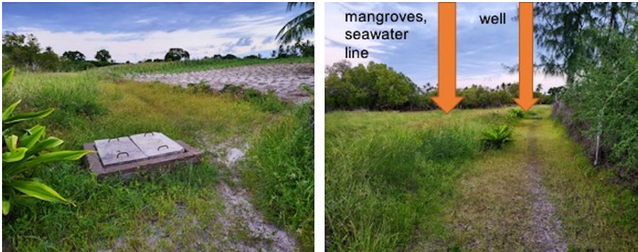
Figure 6. Modern well on the island of Kirepwe in Mida Creek, Kenya. The picture on the right shows that the well is placed just above of the water line at high tide (photos. M. Baumanova).
