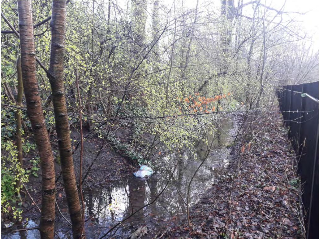
Figure 4: Nico Ditch at Platt Fields, Fallowfield, in February 2020, where it functions as a drainage channel (Photograph: Michael Nevell, 2023)
