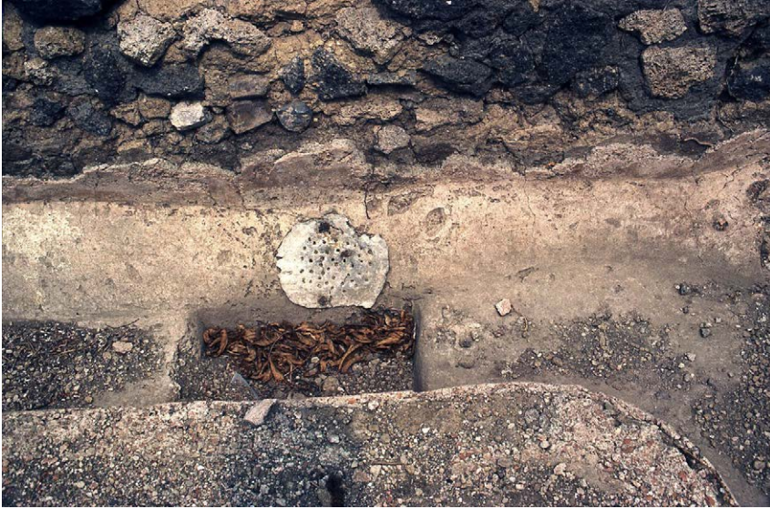
Figure 3. Pompeii, house I 9, 11.12, gutter in garden with access to cistern: a settling basin and in front of the opening to cistern a lead perforated sheet attached with iron nails (photo by the author, published with permission of the Ministero della Cultura - Parco Archeologico di Pompei).
