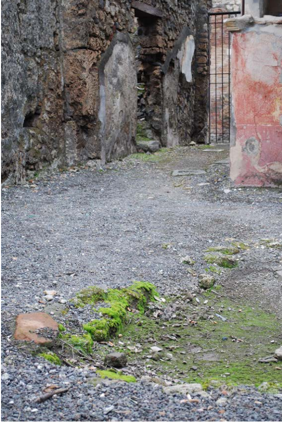
Figure 10. Pompeii, house IX 2, 26, badly preserved impluvium with drain to street visible by two little inspection holes (photo by the author, published with permission of the Ministero della Cultura - Parco Archeologico di Pompei).
