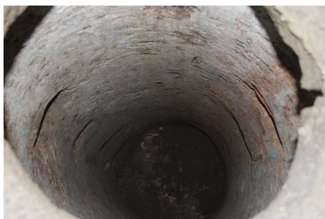
Figure 12. Pompeii, Casa del porcellino (IX 9, c), descending foot holes in cistern shaft (photo by the author, published with permission of the Ministero della Cultura - Parco Archeologico di Pompei).
