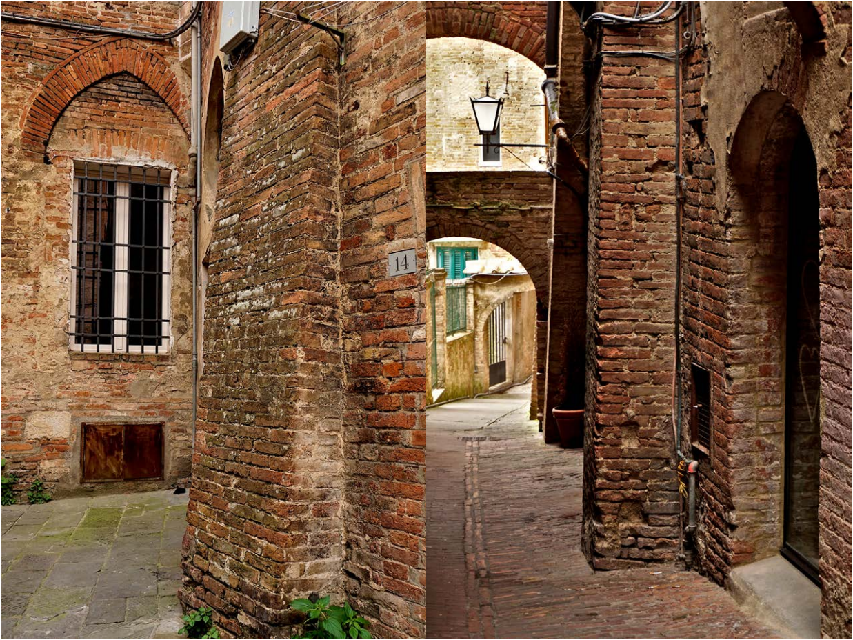
Figure 4.8 - Example of buttresses inserted above wall (Photo: Valeria Razzante)
