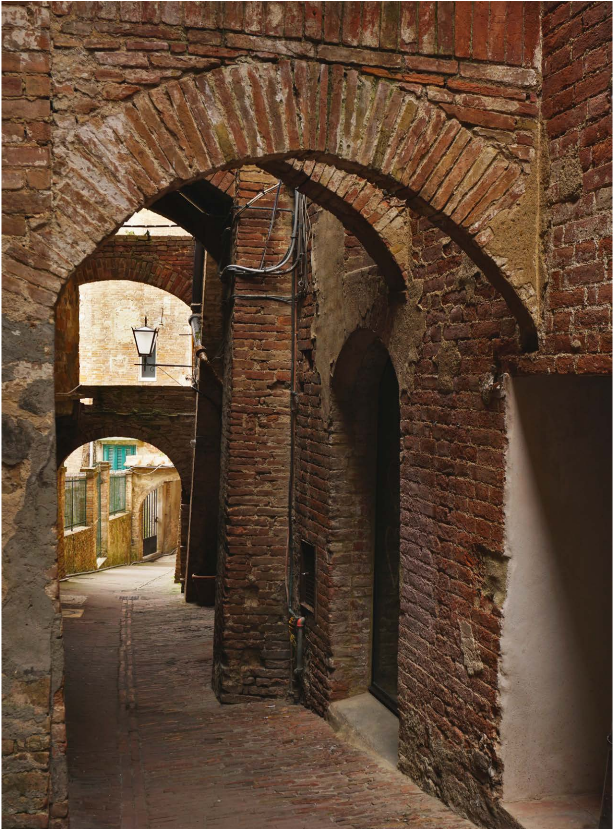
Figure 4.10b - Examples of buttressing arches.
