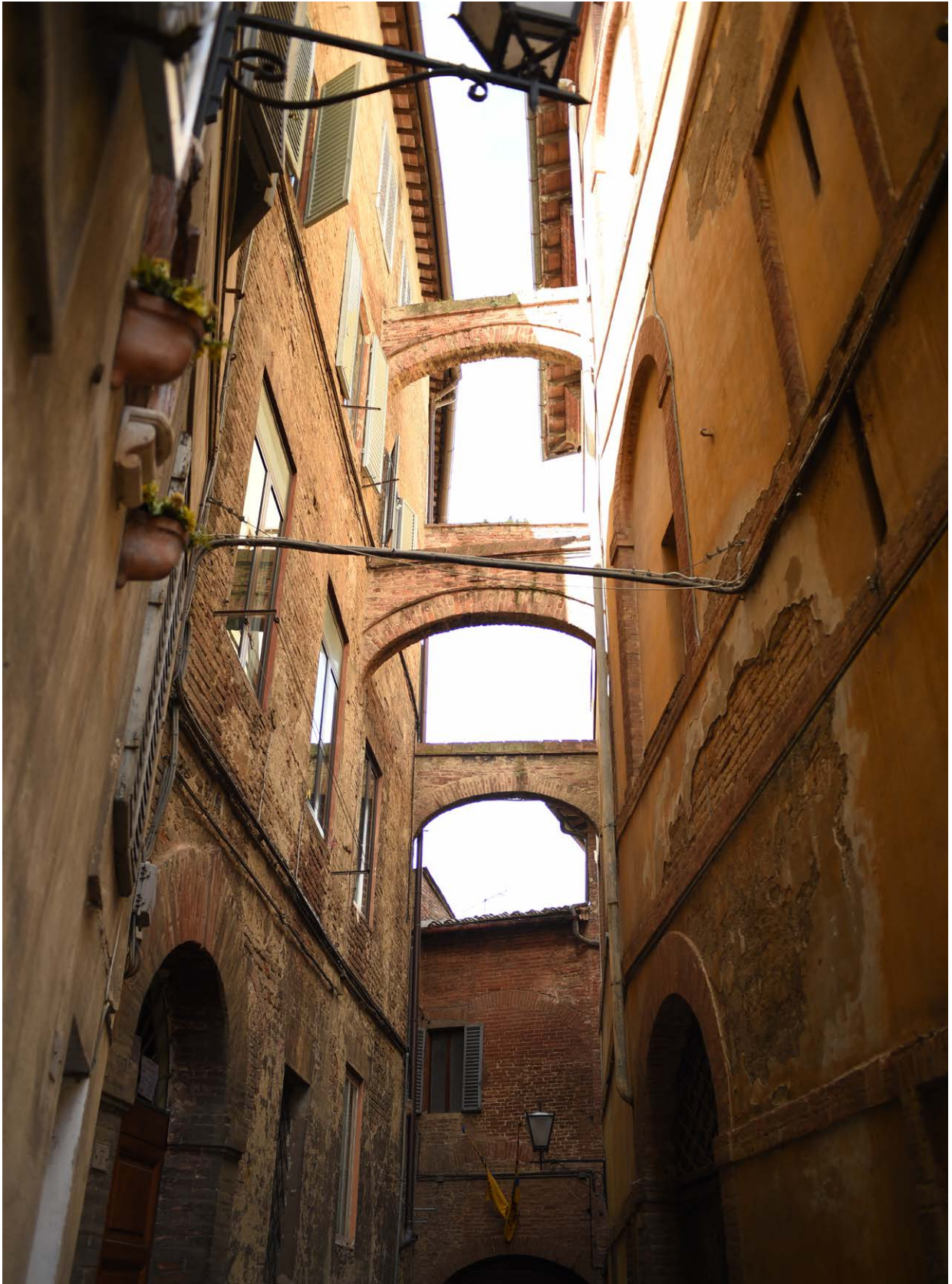
Figure 4.10a - Examples of buttressing arches
