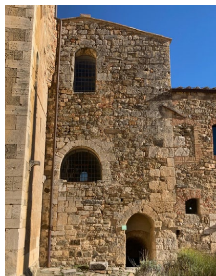
Figure 4.27 - The facade of the sacristy, on the side facing the cloister.
