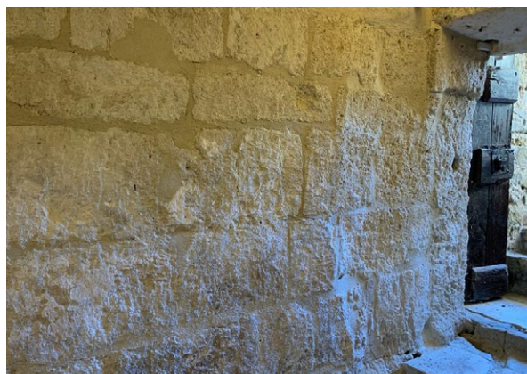
Figure 4.23 - Detail of the masonry technique (with large dressed blocks) in crypt below sacristy. Note absence of breaks in the wall at the point where the doorway is situated, showing that the doorway leading to the sacristy's facade is contemporaneous with this room.
