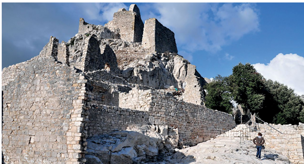
Figure 5.36 - The open space accessed from the main entrance to the castle.
