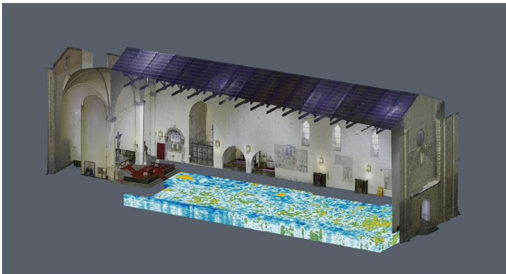
Figure 1 - Digital representation of the church of San Domenico (Città di Castello) with the GPR dataset in point cloud format.
