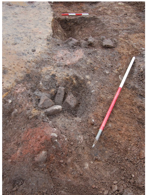
Figure 2.21 Foundation trench [289] of Phase 3 Building 3 (Shot faces southeast, 40cm and 1m scales).
