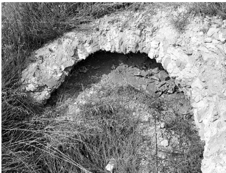
Figure 202. Vault over inner circular corridor seen from above (1981).
