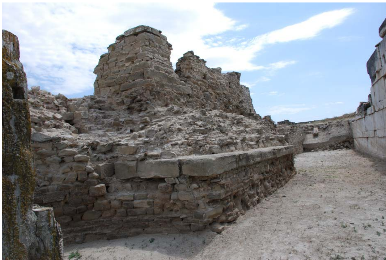
Figure 70. West Porch looking west, Phase I.
