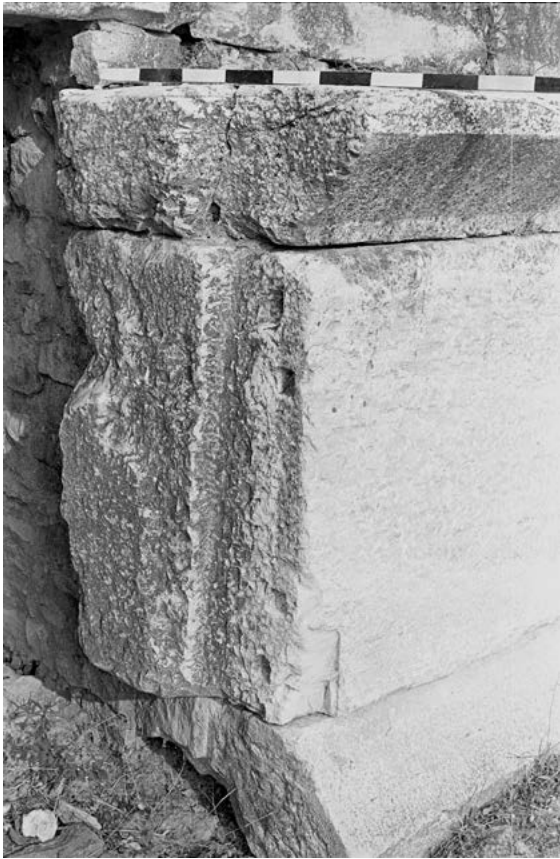
Figure 258. West refuge, north side of entrance.
