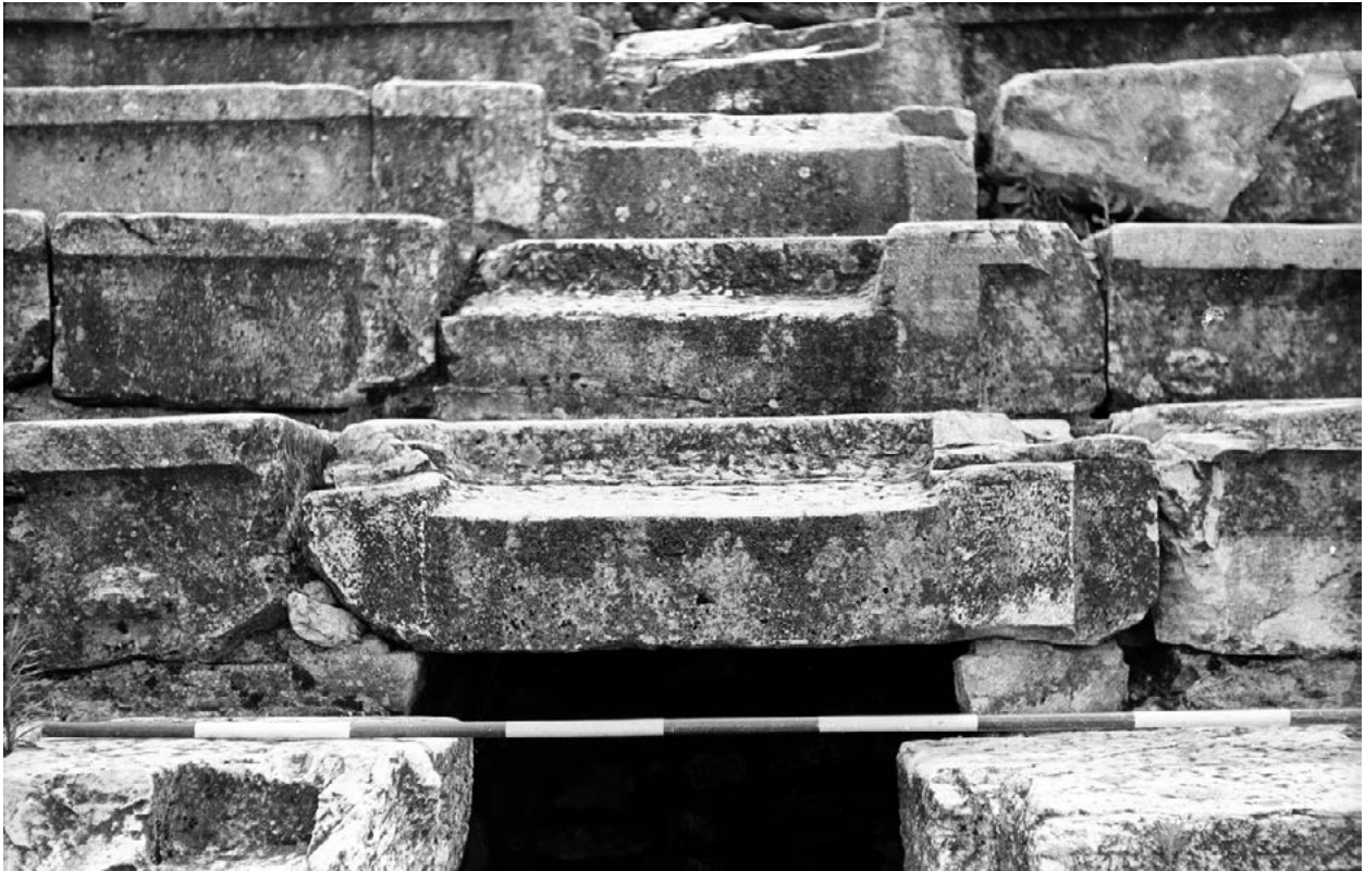
Figure 254. Stair 2, rows 1-4 above west refuge.
