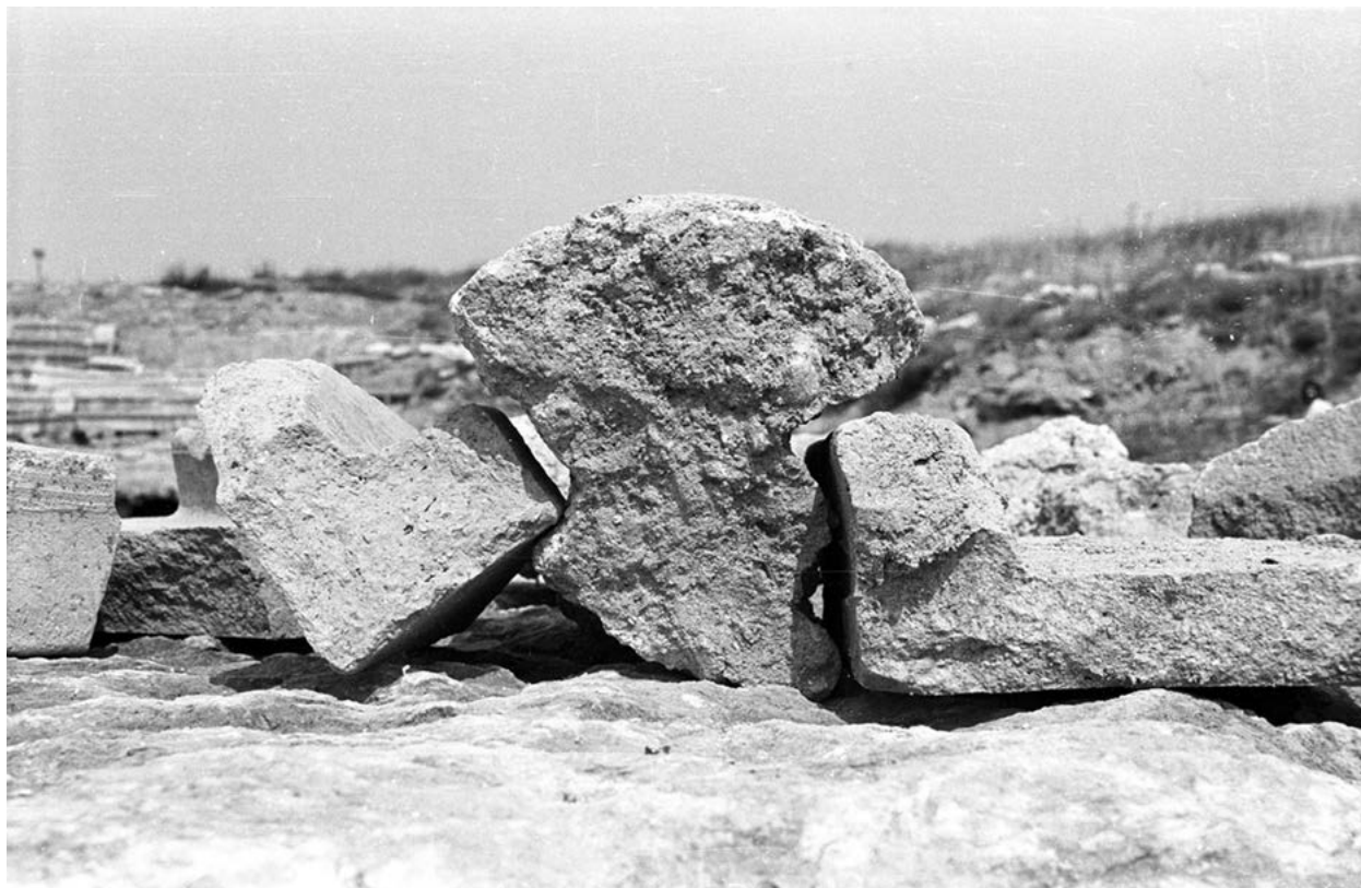
Figure 80. Two flat pan tiles with the mortar bedding for a curved cover tile from destruction debris from the roof, Phase II.
