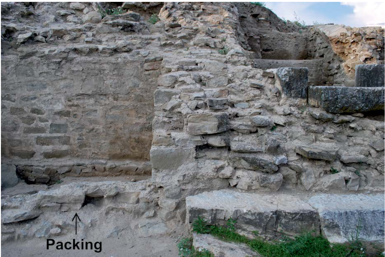
Figure 17. First phase wall 9 and east additus = East radial corridor, Phase I, first circular wall at left bonded to wall 9.
