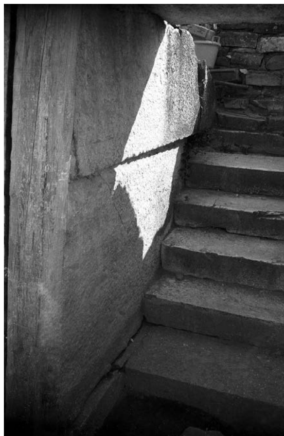
Figure 200. Stairway to seats, west radial corridor.
