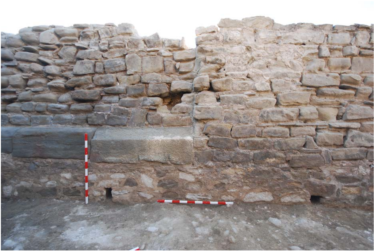
Figure 26. Wall 6 of east additus maximus, looking south = East Radial Corridor.
