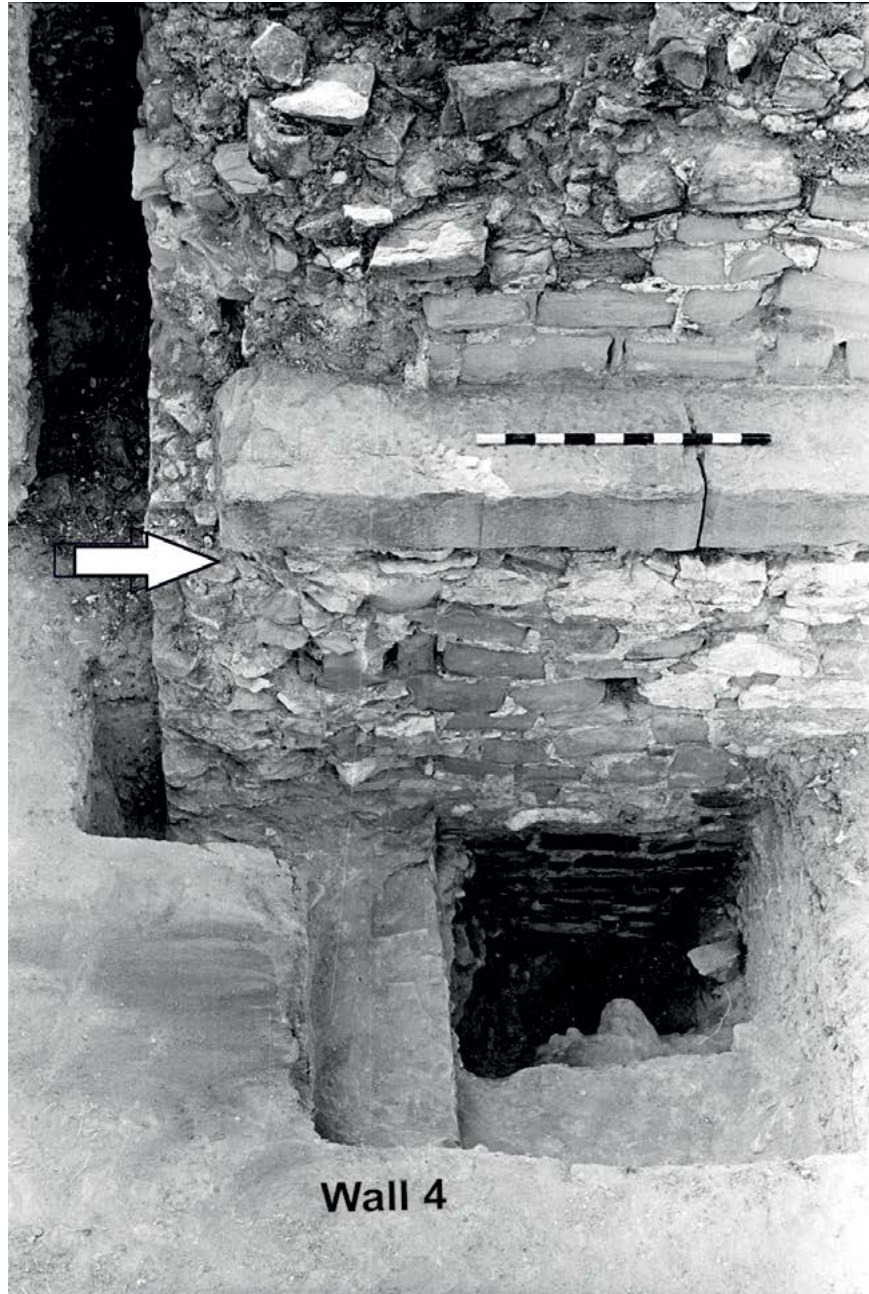
Figure 38. East end of East Porch showing rough surface on north face after wall 4 was dismantled. Remains of wall 4 below. Note: scaffolding hole. Trench XXV in foreground.
