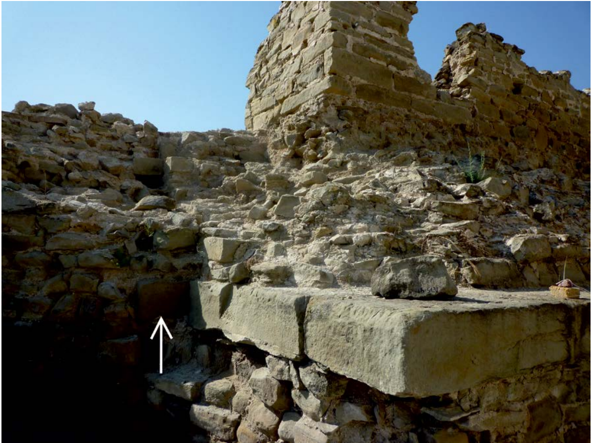
Figure 48. Return of green course at east end of West Porch.
