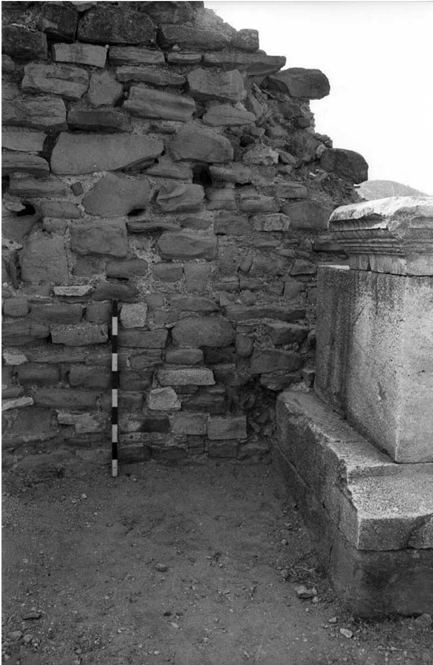
Figure 93. East Porch III and east bay of East Paraskenion, looking south.
