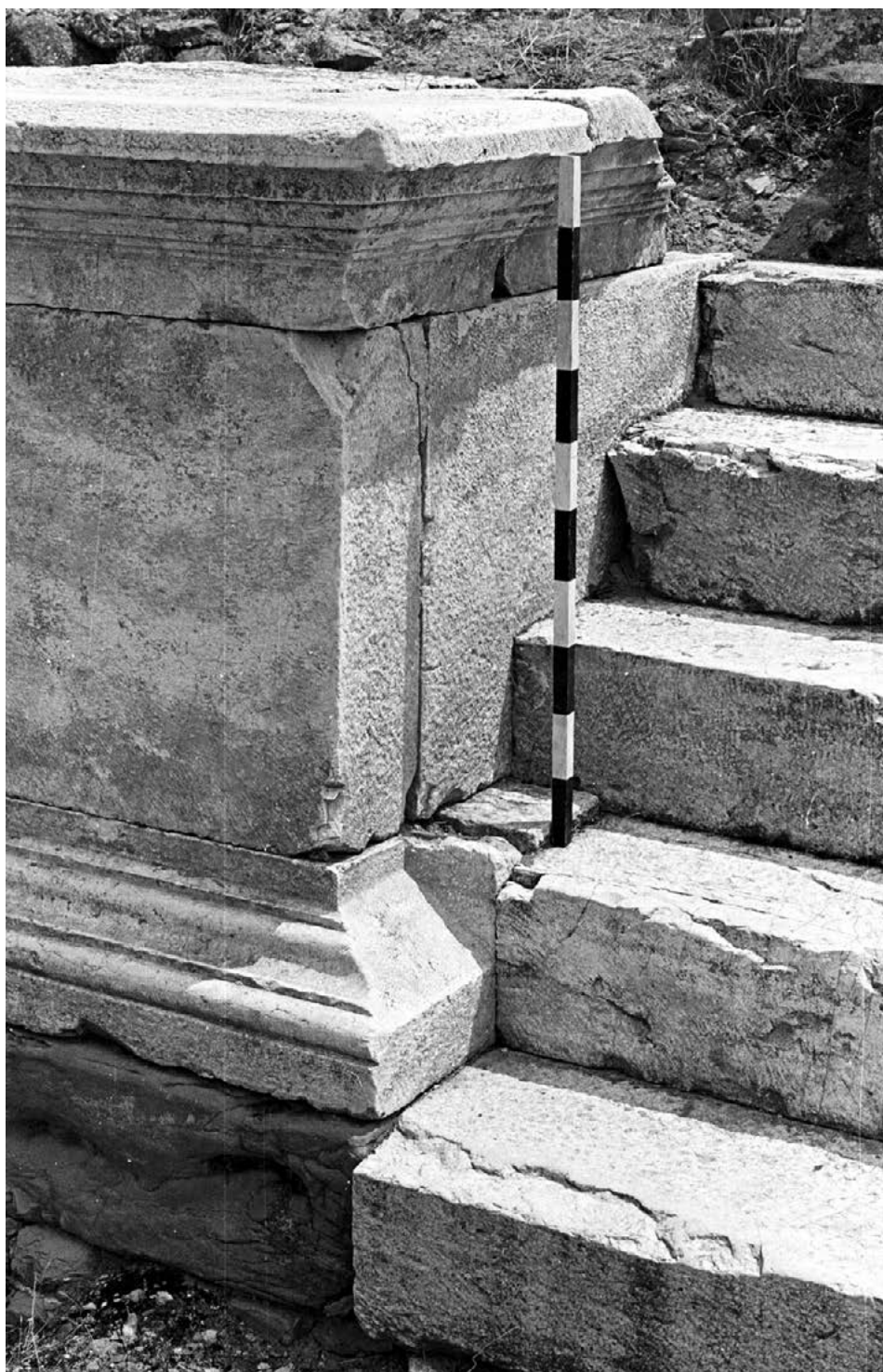
Figure 85. East Porch II and East Stair I.
