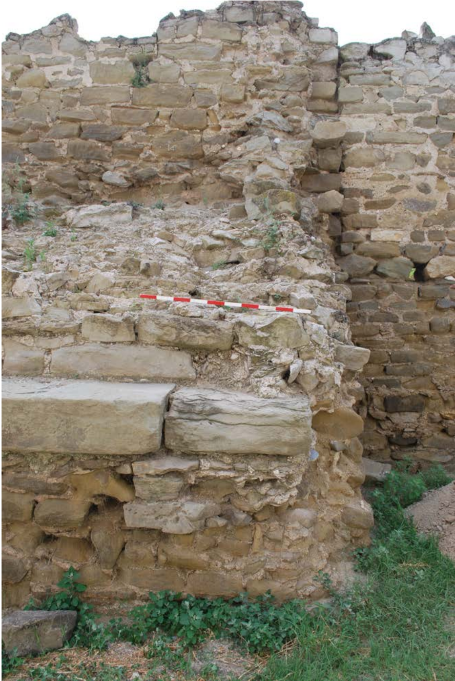
Figure 39. West end of West Porch. Note: rough surface where wall 2 removed.
