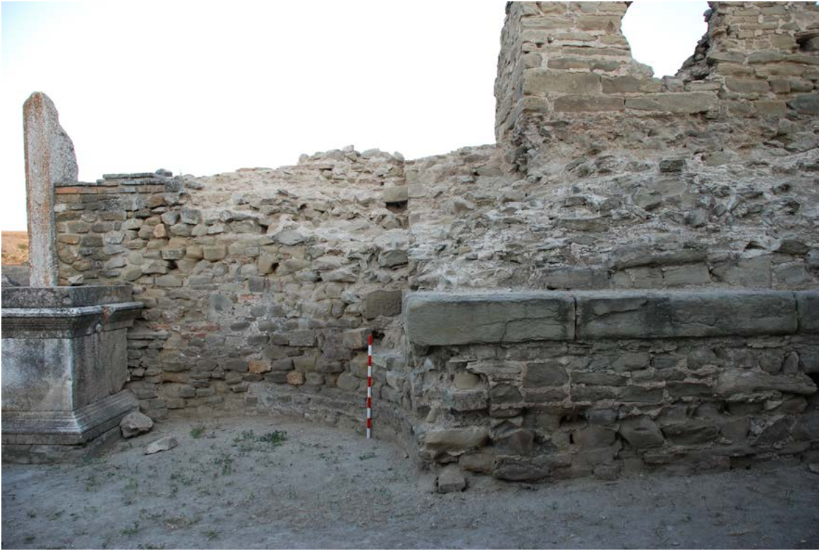
Figure 42. East end of West Porch, looking south. Phase I.
