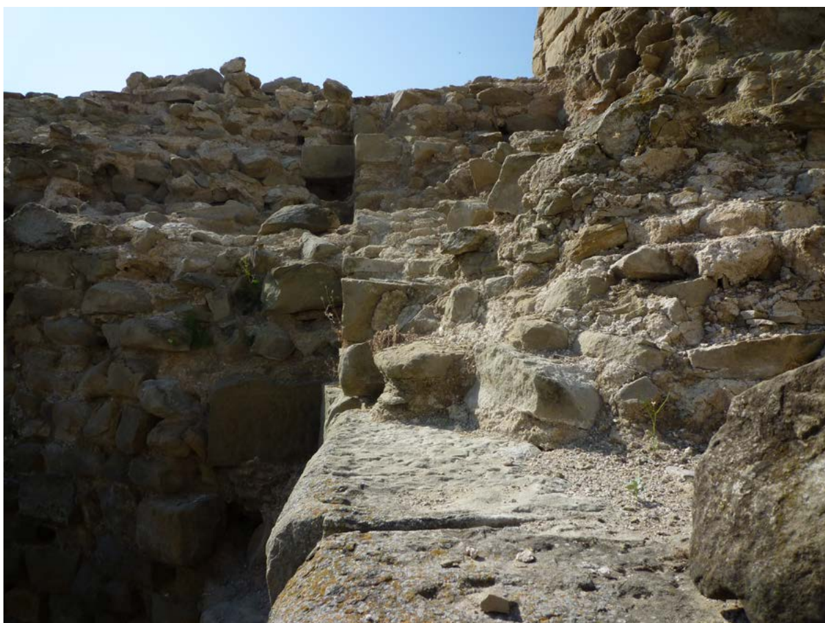
Figure 55. Return of front wall, along West Porch, Phase I, looking south.
