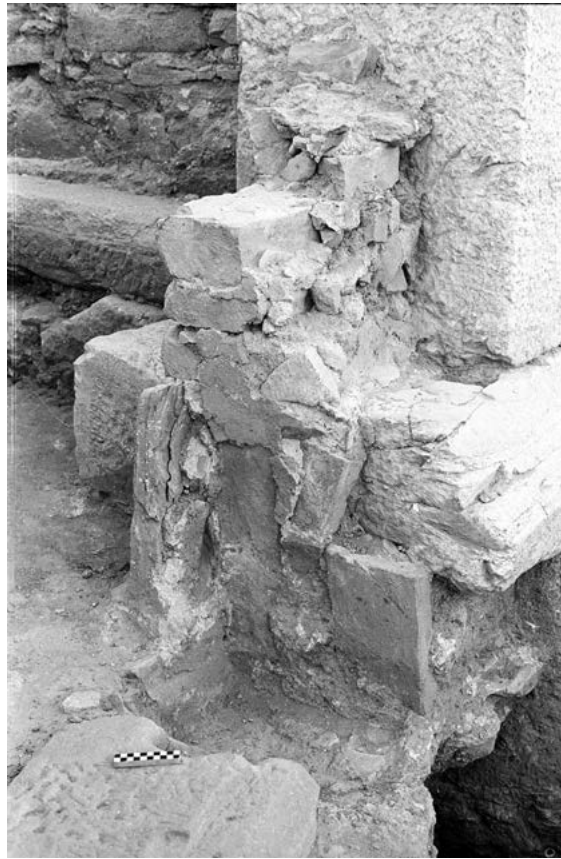
Figure 259. Center refuge, east side of entrance, door jamb of Phase III (1974).
