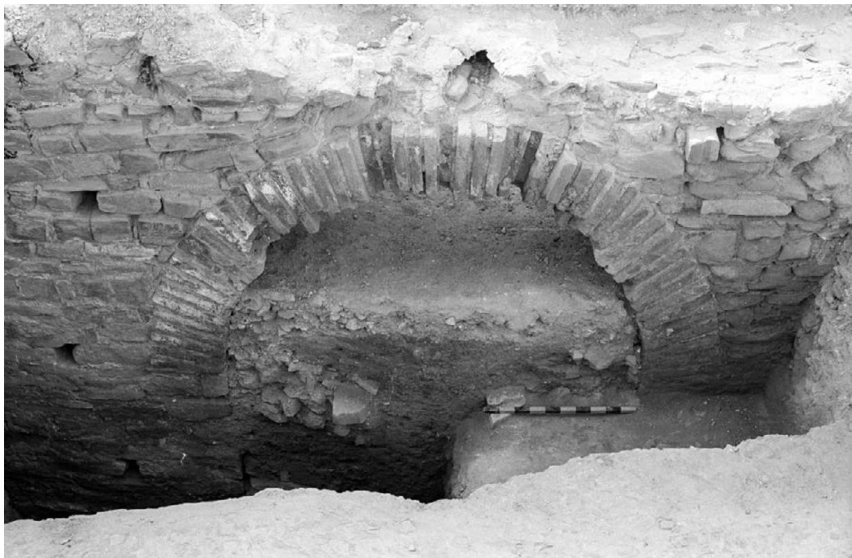
Figure 198. Center radial corridor at junction with outer circular corridor, looking north.
