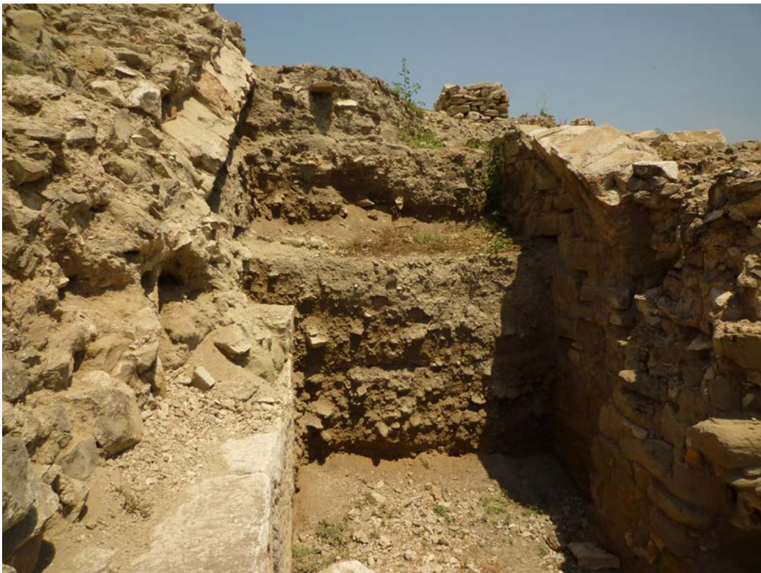
Figure 161. East additus maximus = east radial corridor vault from looking east.
