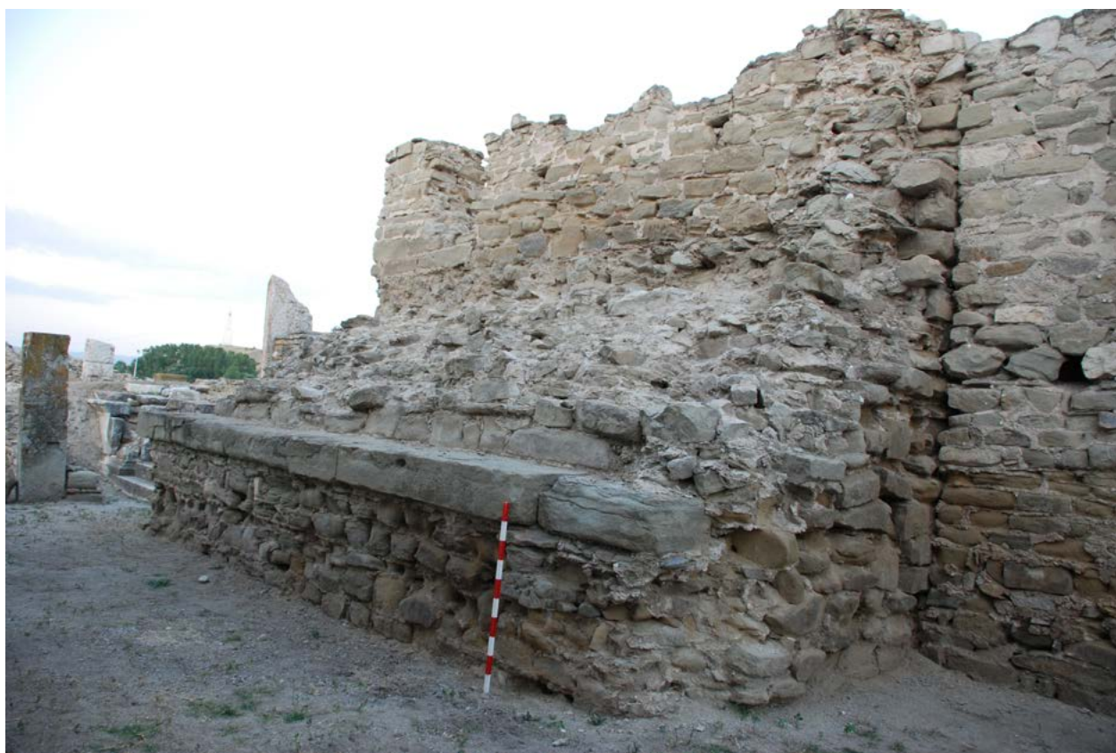
Figure 40. West Porch, entire. Phase I.
