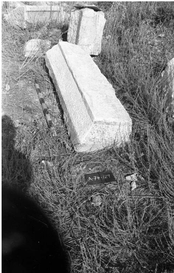
Figure 182. No. 2 base course.
