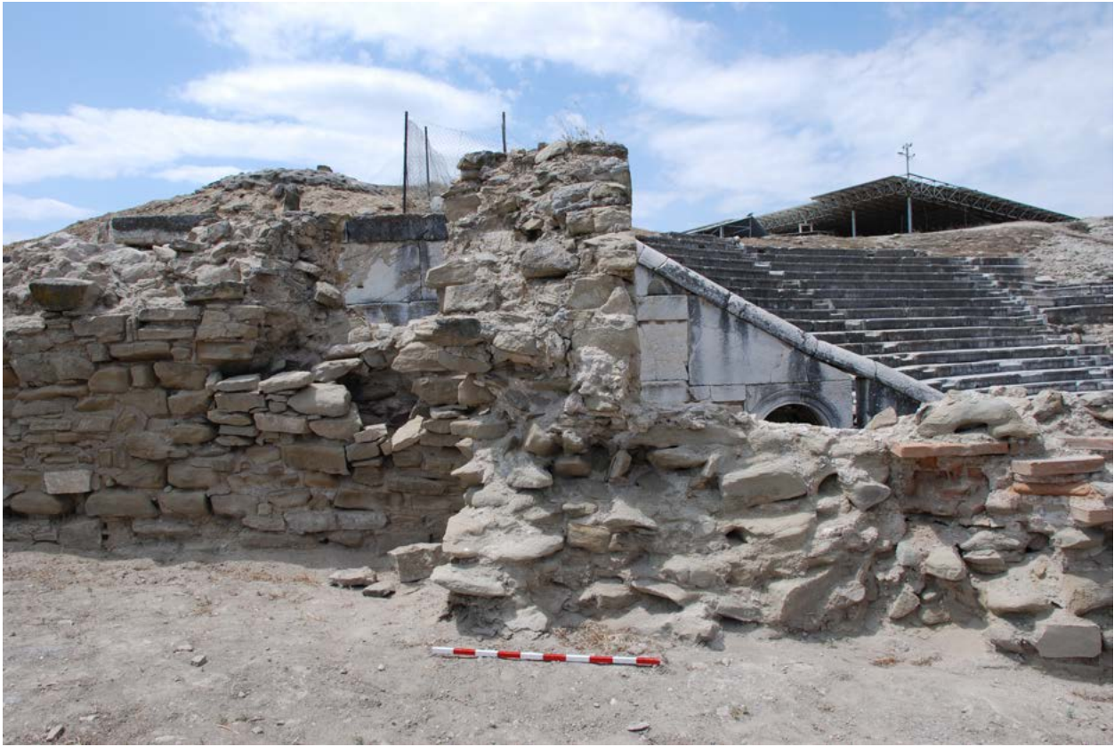
Figure 46. Remains of front wall, Phases I and II looking north, 2009.
