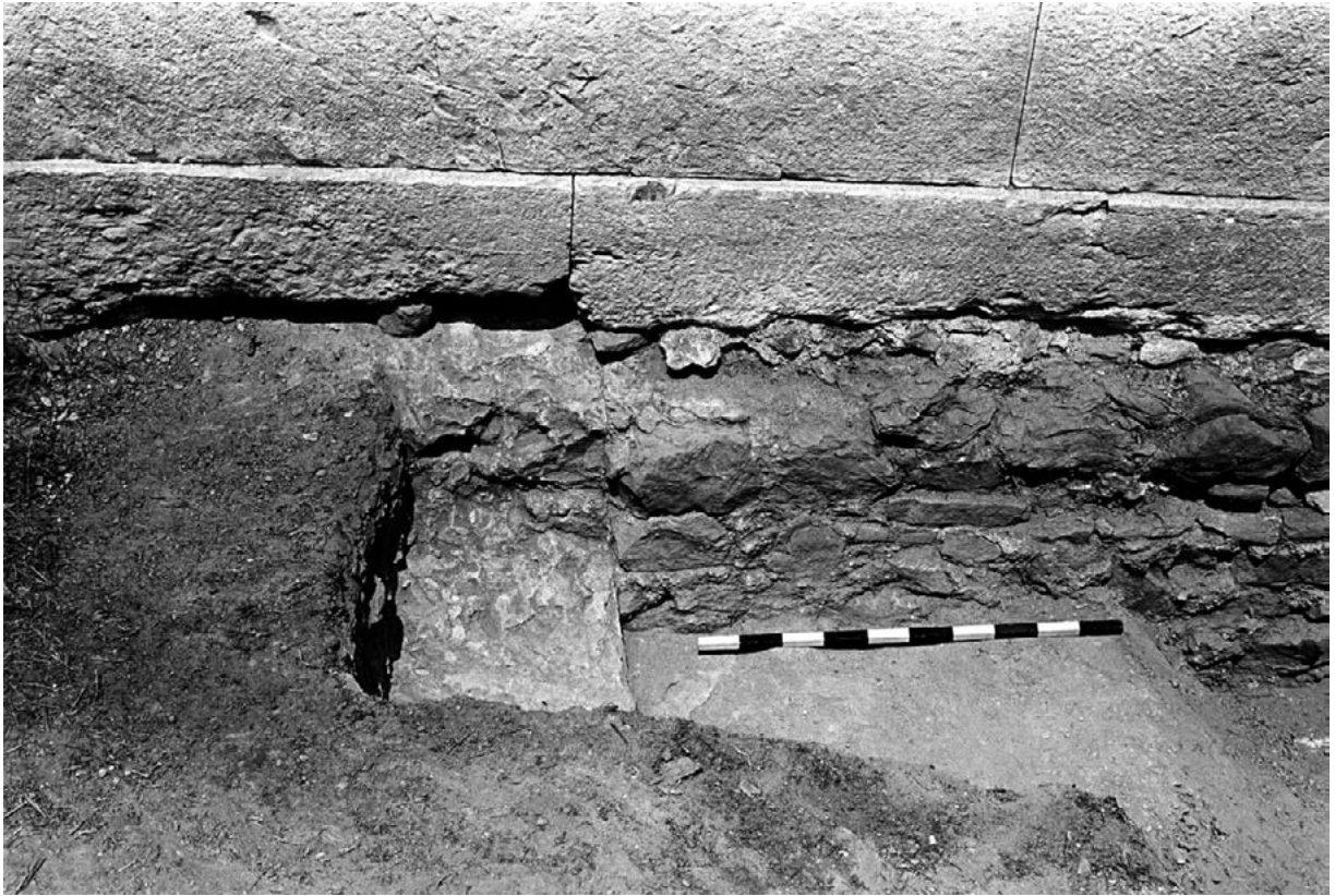
Figure 205. Foundation and base course of east analemma built over north end of Phase I wall 4. Trench XXV in foreground.
