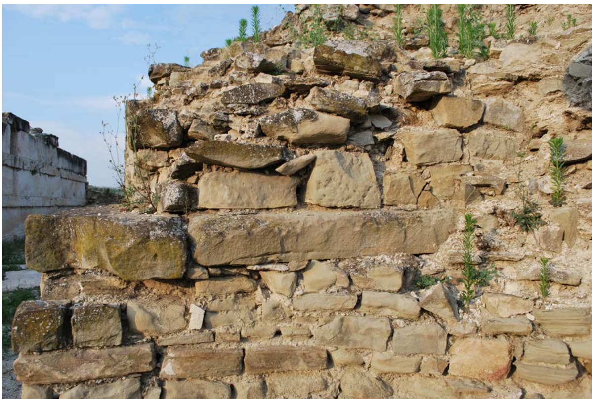
Figure 54. West face of East Porch, green course return, Phase I.
