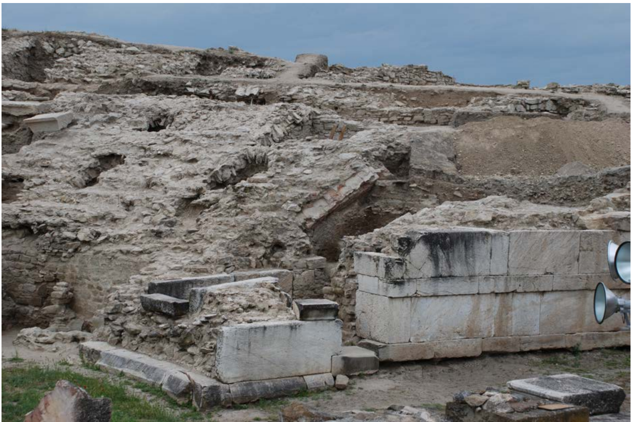
Figure 204. General view, east cavea seat foundations after excavation and before restoration, looking northeast.
