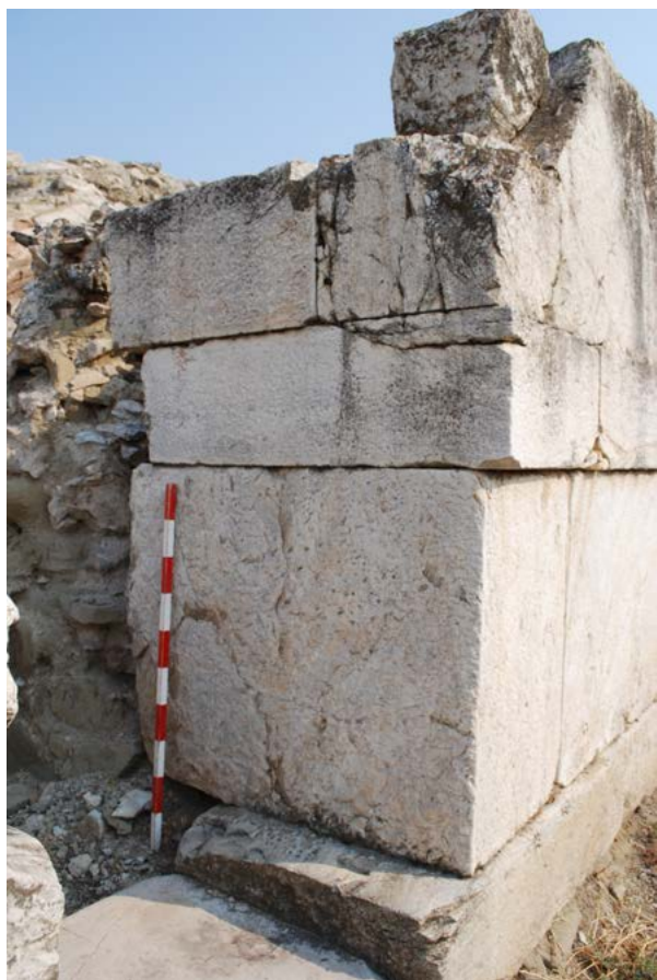
Fig. 199. Doorway to east anteroom.
