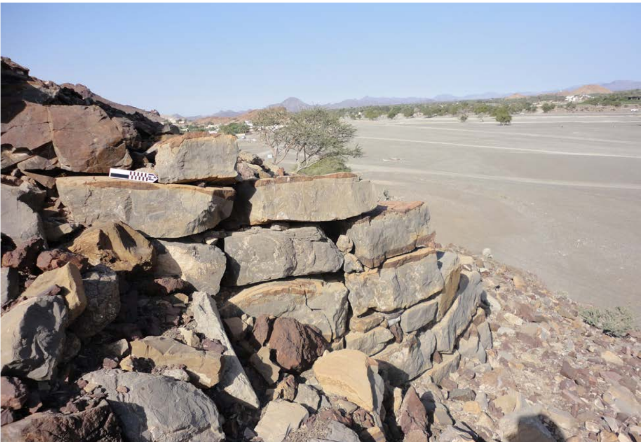
Figure 1.34. The tower Abu Suwaih B overlooking the wadi (photograph by ArWHO, used with kind permission).
