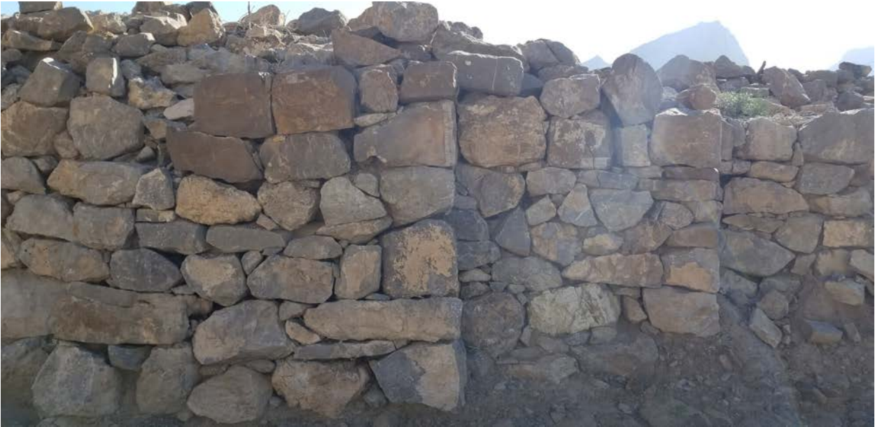
Figure 1.23. Close-up of the exterior wall elevation showing the “stepped” construction technique.
