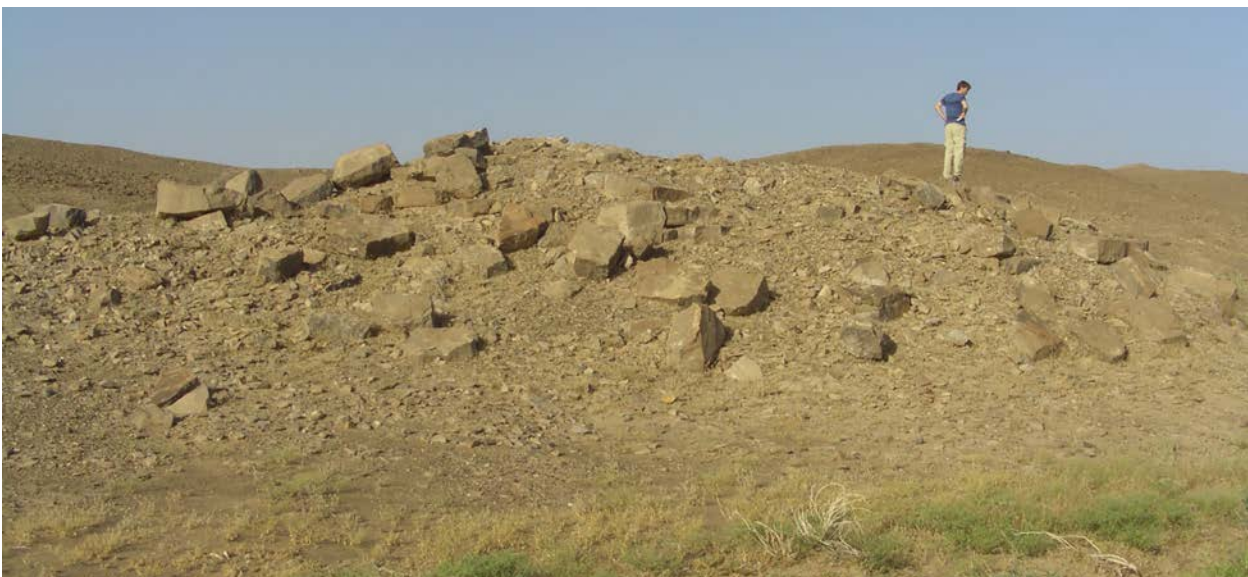
Figure 1.65. View of Al-Araqi tower.
