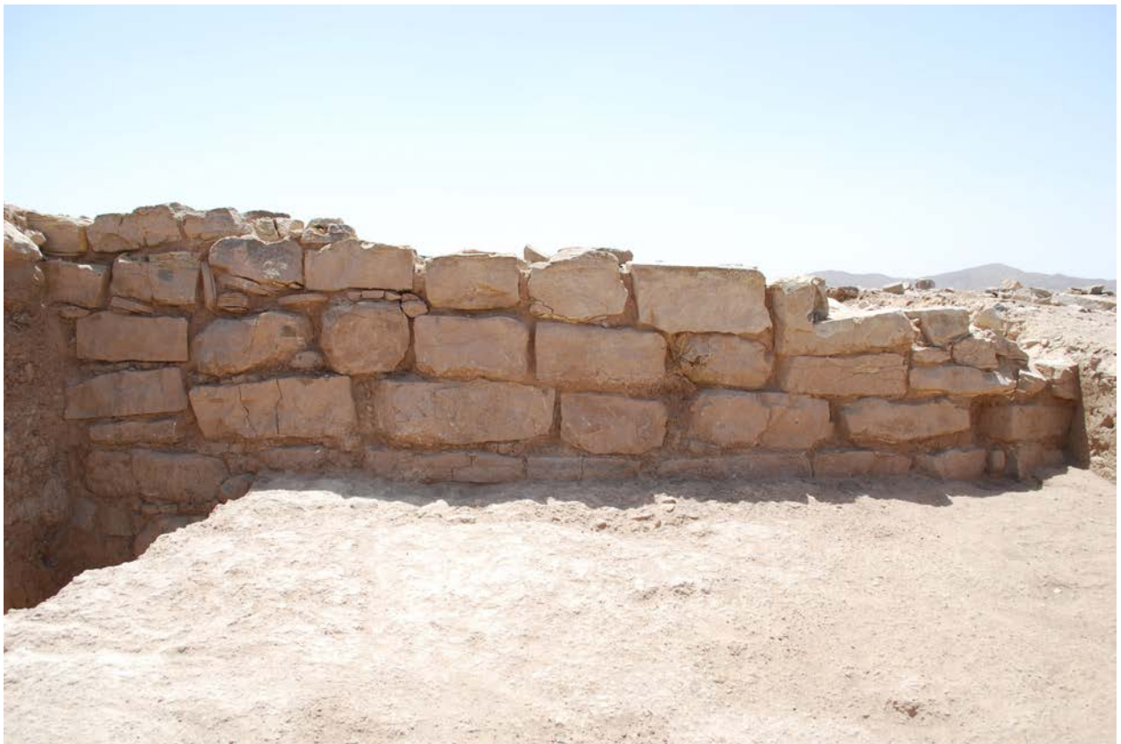
Figure 1.85. Ringwall of Building II at Bat.
