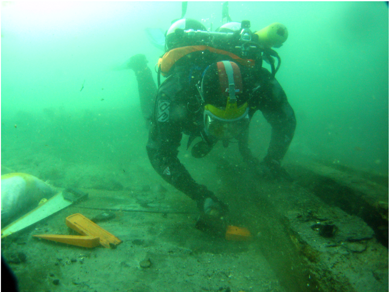
Figure 2.9. Dismantling the timbers underwater
