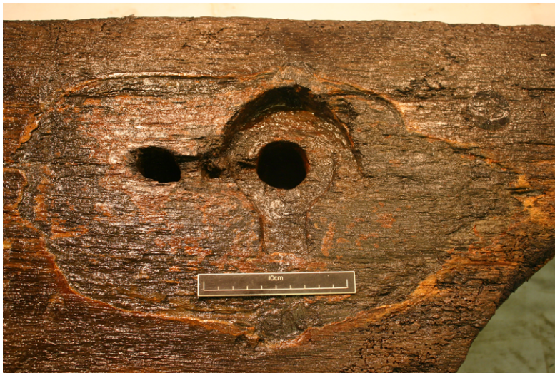
Figure 4.54. Recessed bolt on the outboard face of SCW1275
