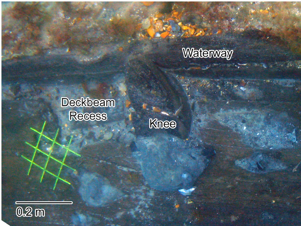
Figure 4.6. Small knee in the stern supporting the quarterdeck
