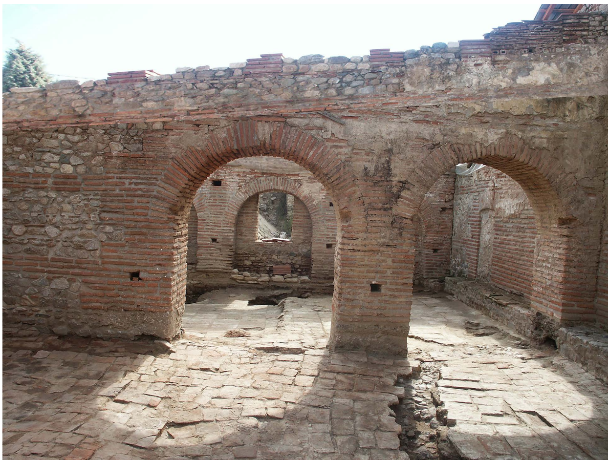
Figure 10. The communication between the frigidarium and the apodyterium. Photo: by Author.
