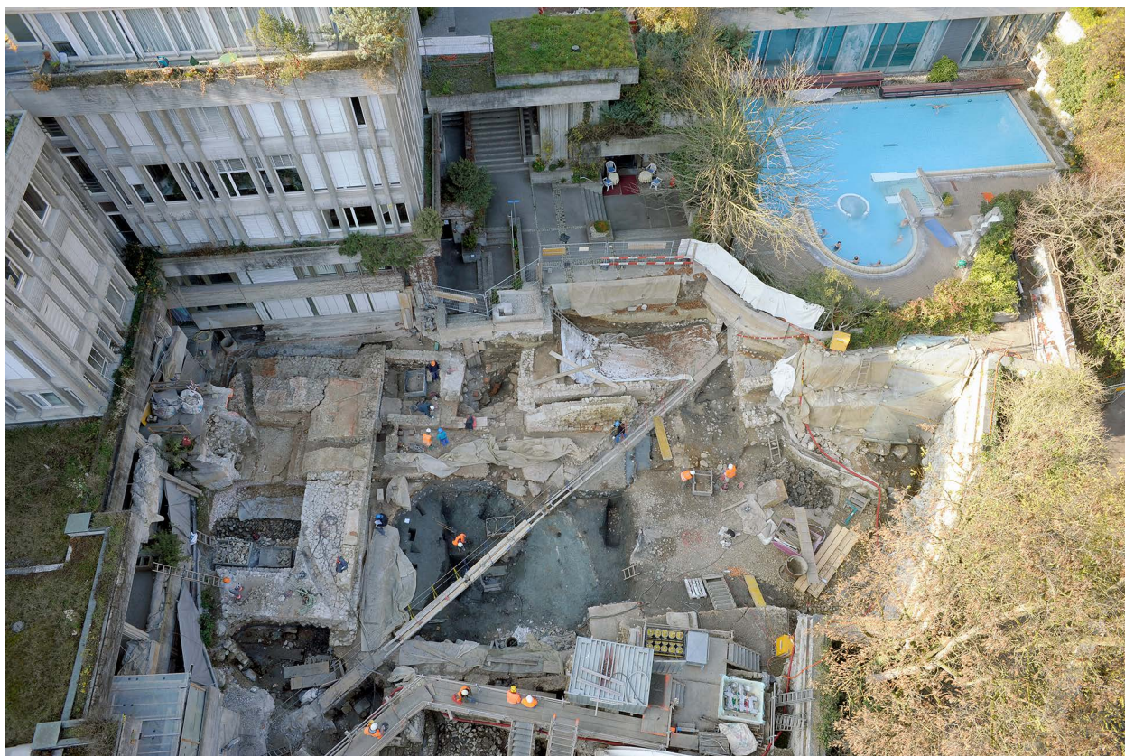
Figure 3. 2000 years of bathing history in Baden. Excavation of the Roman thermae, while the old brutalist public thermal bath is still use in 2011. © Photograph Archaeological Service Aargau/Samuel Mühleisen.
