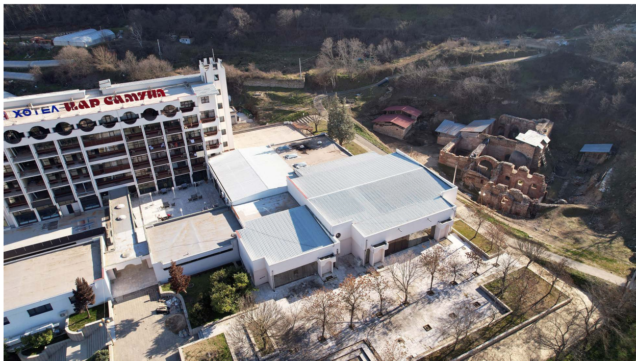
Figure 11. Car Samuil Hydrothermal Medical Center, sited close to the Roman thermal spa. Photo: Aleksandar Donchev.
