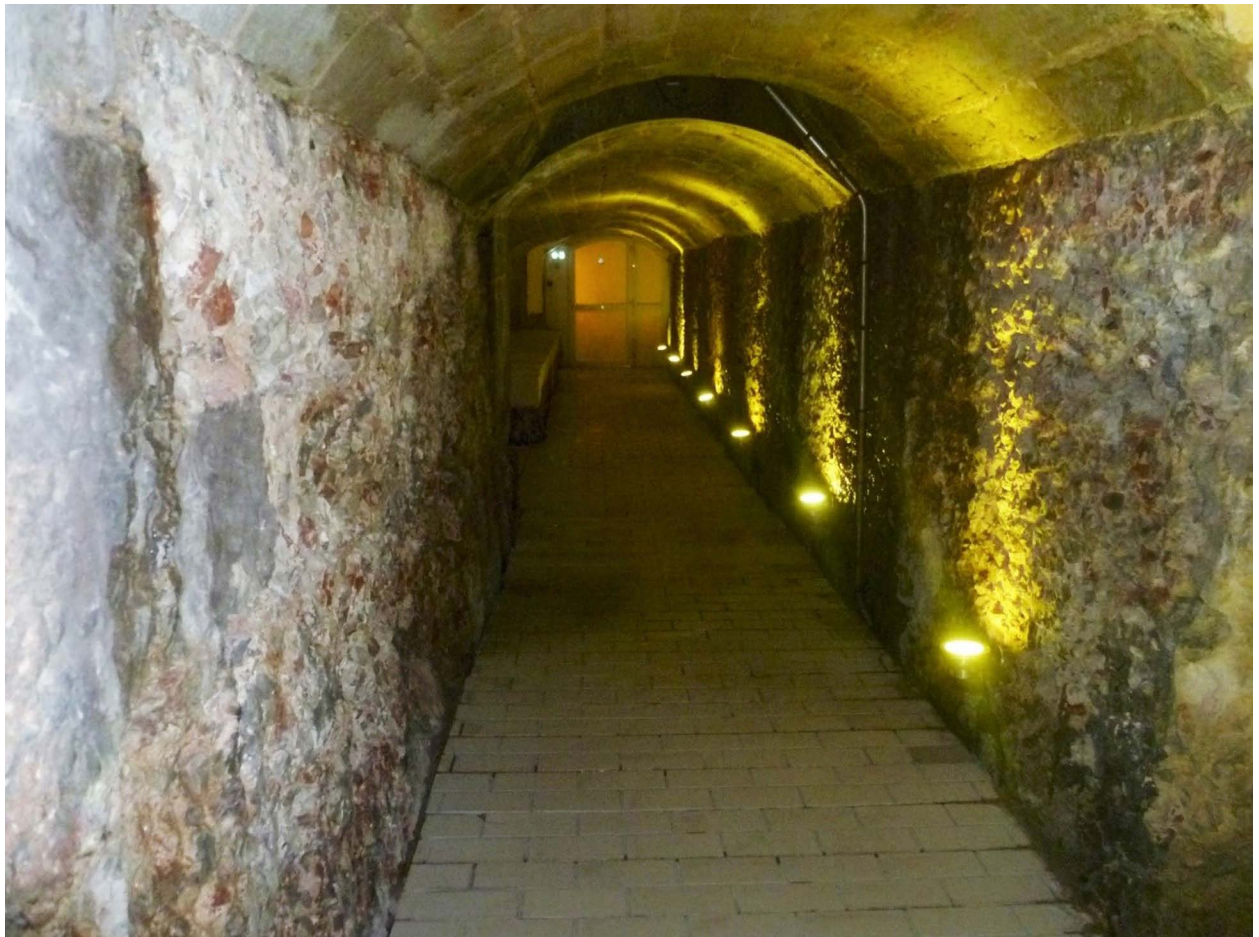
Figure 6b. Photo of the Jutier corridor in Plombières-les-Bains, excavated in the Roman opus caementicium slab (photo by https://remiremontvallees.com/2019/06/12/plombieres-les-bains-et-ses-vestiges-antiques/ , viewed 12 th June 2019).
