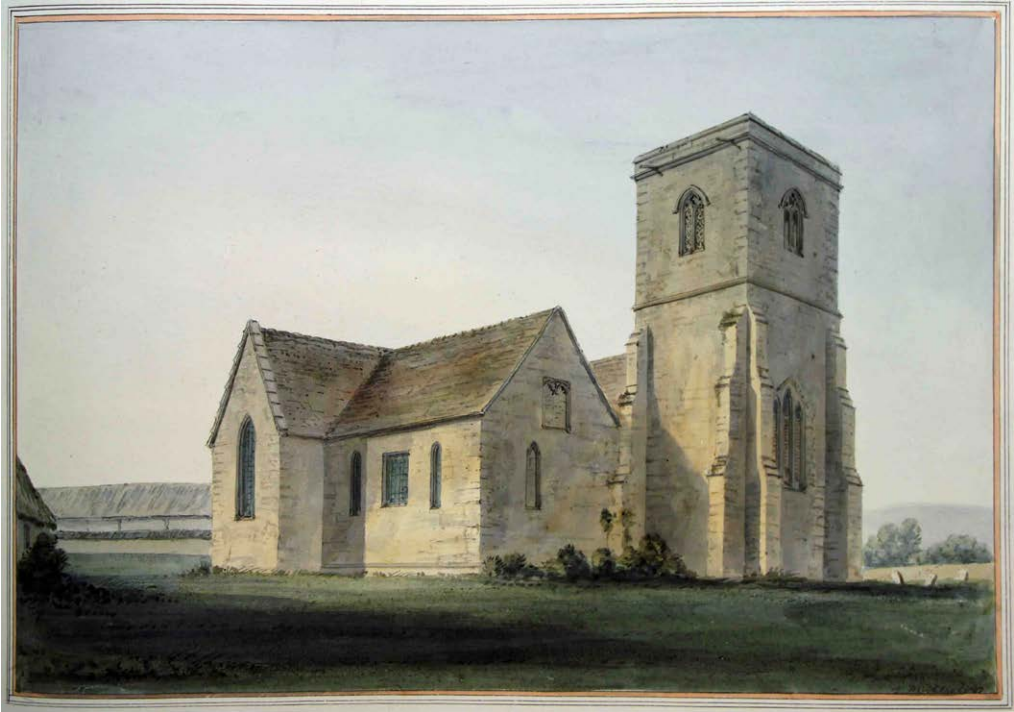
Figure 11.6: Fisherton Anger church from the North West, 1803, by John Buckler. © Wiltshire Museum, Devizes [accession no., DZSWS:1982.356].
