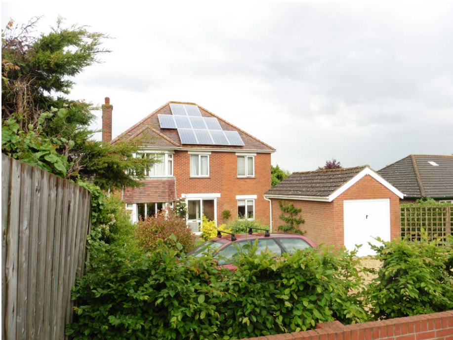
Figure 13.21: Private house in Milton Road. Originally built c.1950, it was expanded (right hand side) in the 1970s (© The Author)
