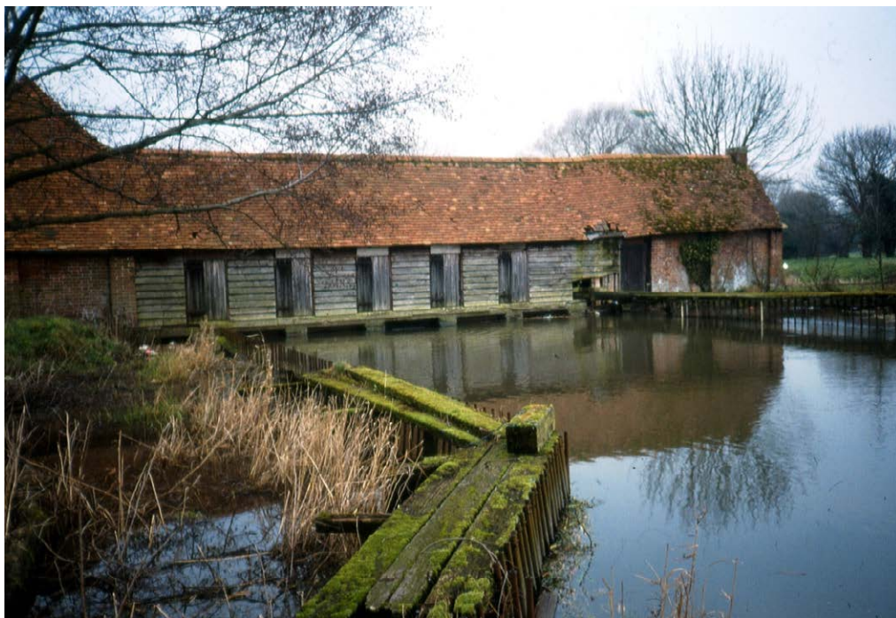
Figure 12.17: Hatch House and Eel Trap (SU 1521 2903) in May 2013
