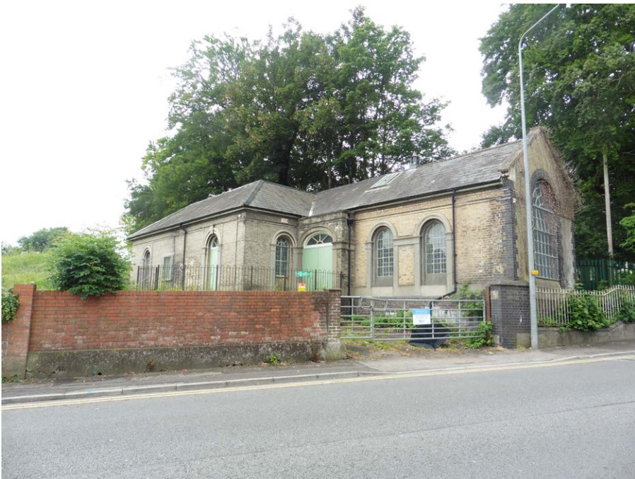
Figure 13.14: The Waterworks and pumping station on Devizes Road. (© The Author)
