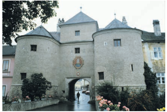
23. The east-gate of the Roman fort at Traismauer on the Danube (Austria) dates to the 4th century but qualifies for nomination under the proposed definition
