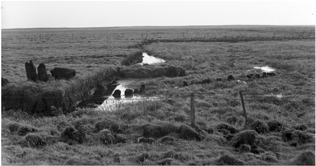
Figure 3 (above): Palisade on the meadow south of Olmersvej looking towards the Tinglev Lake (Photograph: Hugo Matthiesen from 1928)
