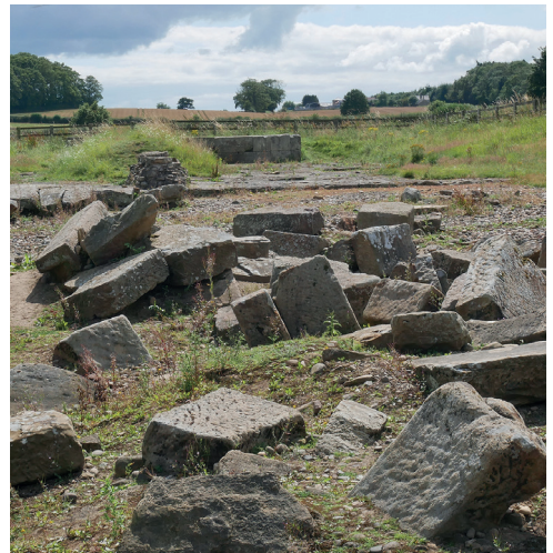
128. The tumbled stones of the bridge at Piercebridge with a surviving pier in the background
