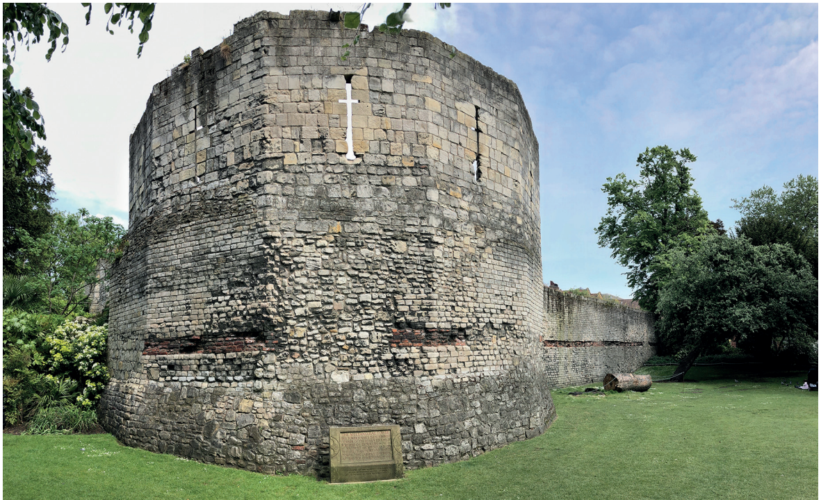
116. The multangular tower at York was one of series of bastions added to the fortress wall at York; the smaller lower stones are Roman
