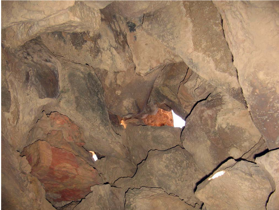
Figure 4.9. View from inside cairn of corbelled walls and capstone roof (photo: Yaqoub Al-Rahbi, Courtesy of Mohamed Al-Belushi, Sultan Qaboos University)
