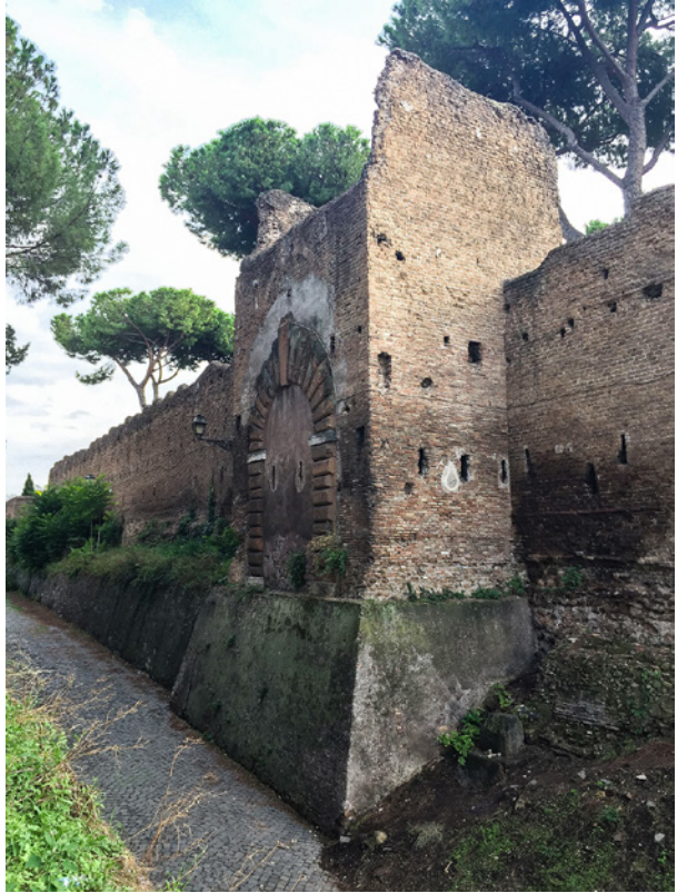
Figure 7. The gate tower (BC1), along the north-east side of the fortress.
