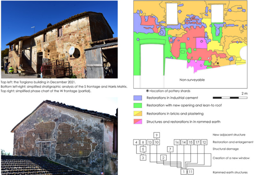
Figure 2 (a-d). The Torgiano farmhouse (stratigraphic details, Harris matrix and relevant building phases).
