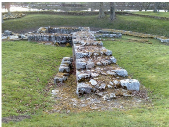
87. The Wall at Chesters bridge abutment showing the earlier foundation to the south
