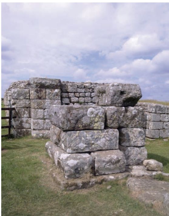
89. The west gate at Housesteads with the upper stones less well dressed than those below
