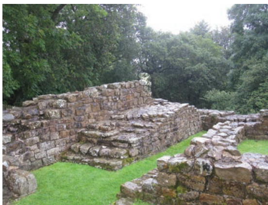
92. The steps which led to the top of the Wall at milecastle 48 (Poltross Burn). But did they lead only to a tower over the north gate or to a wall-walk?
