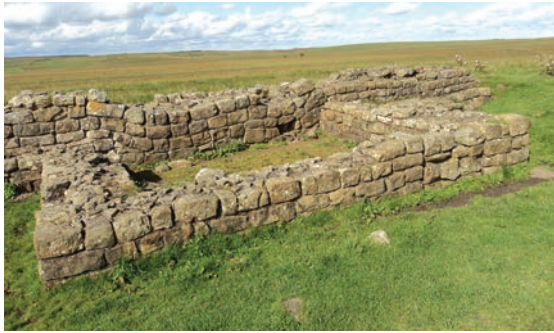
98. Turret 33b (Coesike) was demolished in the late second century
