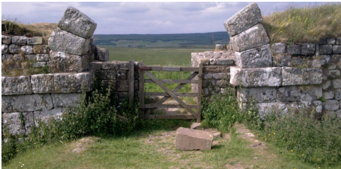
124. The north gate of milecastle 37 (Housesteads)
