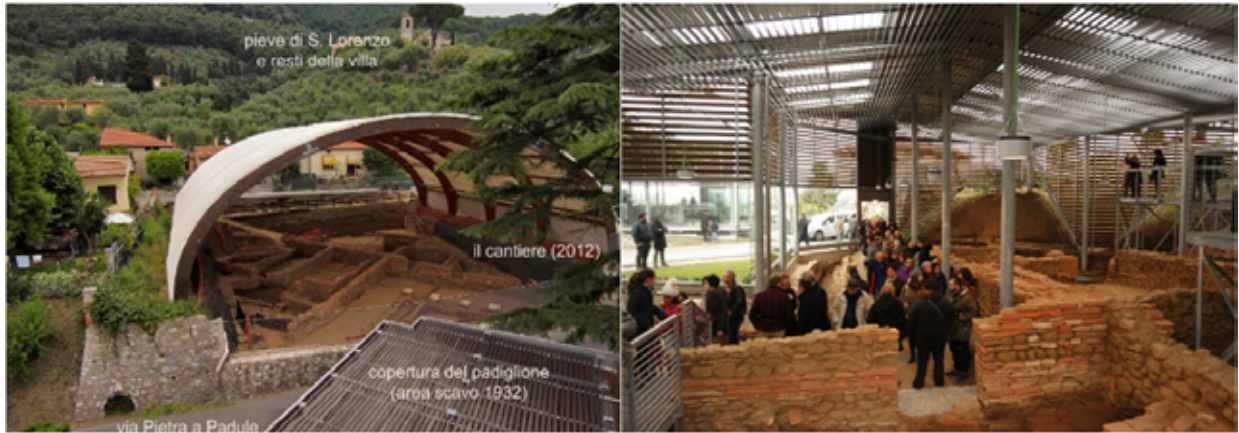
Figure 4.3: On the right, the temporary structure covering the building on the upper part of Via Pietra a Padule during excavation (Anichini et al. 2012, p. 31); on the left, the new pavilion “Il Cantiere”, on the inauguration day (photo: Giulia Osti).
