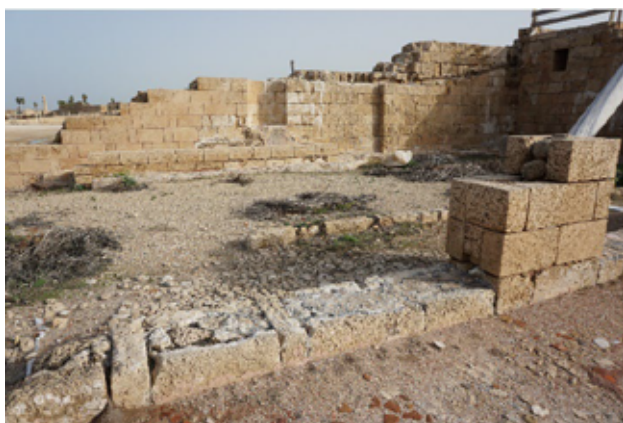
Figure 30. Low Garden compartments G1, 2, 3 and fountain G4, view to the north-east (P. Gendelman).
