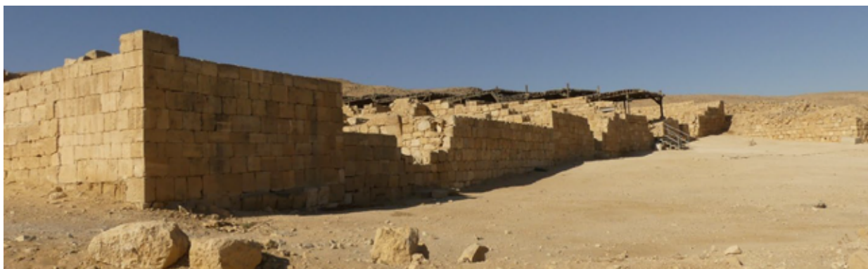
Figure 12. Northern wall of army camp and commander residency (photo O. Sion).
