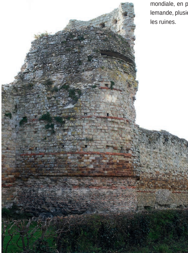
143. Semi-circular bastion at Pevensey. The upper part was added during World War II. The horizontal slot accommodated machine-guns
