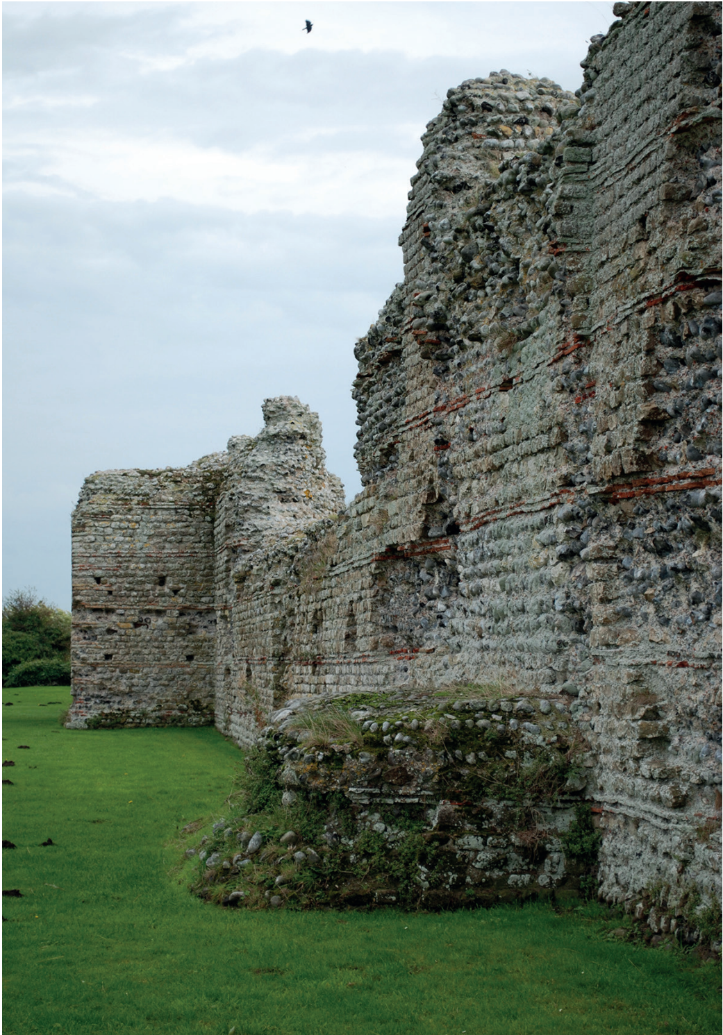
111. The north wall of Richborough fort from the west showing a robbed interval tower, and the tower incorporating the northern postern gate
