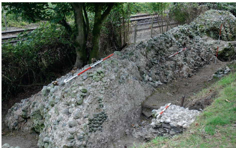
113. The collapsed east wall of the fort of Richborough Le mur est, effondré, du fort de Richborough
