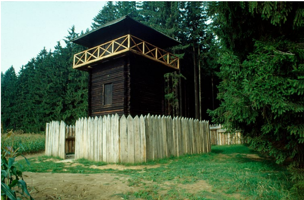
Figure 50. The timber tower at Mahdholz recently created, one of the many treats provided by the Denkmalpflege in Baden-Württemberg
