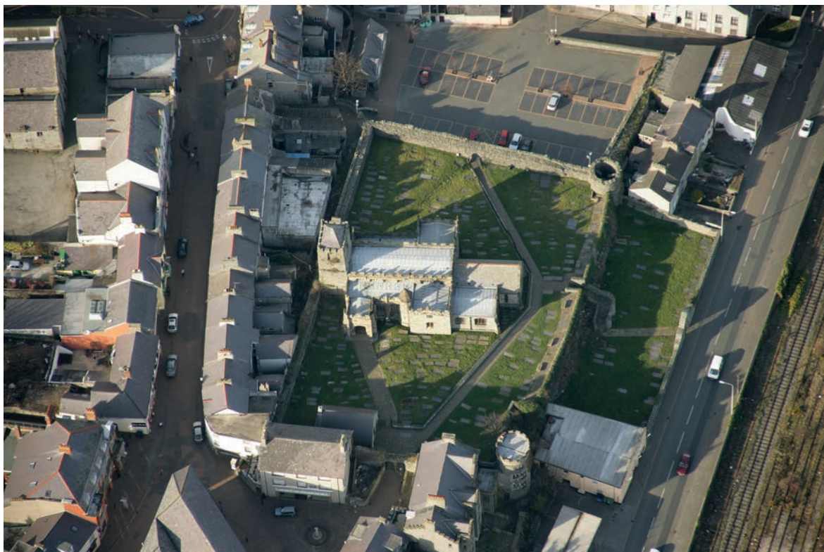
122. Caer Gybi: The Late Roman fort at Caer Gybi overlooking Holyhead harbour. The stout walls enclose the church of St Cybi
