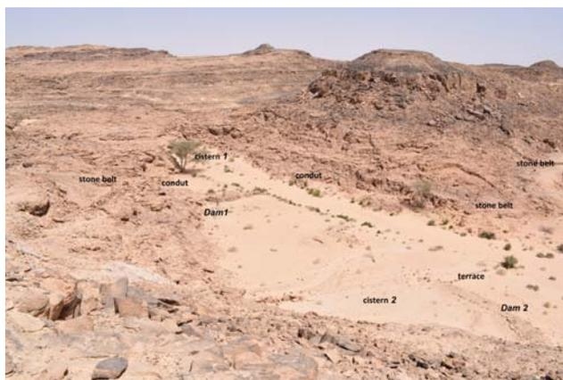
Figure 2. Constructions for collecting run-off water, in the valley's north-east tributary.
