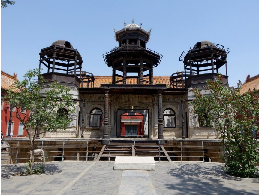
Figure 1. Frontal view of the Lingzhao Pavilion. Part of the marble base that is above the ground can be seen. The central octagonal pavilion and the hexagonal towers to the southeast and southwest are clearly visible. Photograph taken by Xiao Litong in May 2020.
