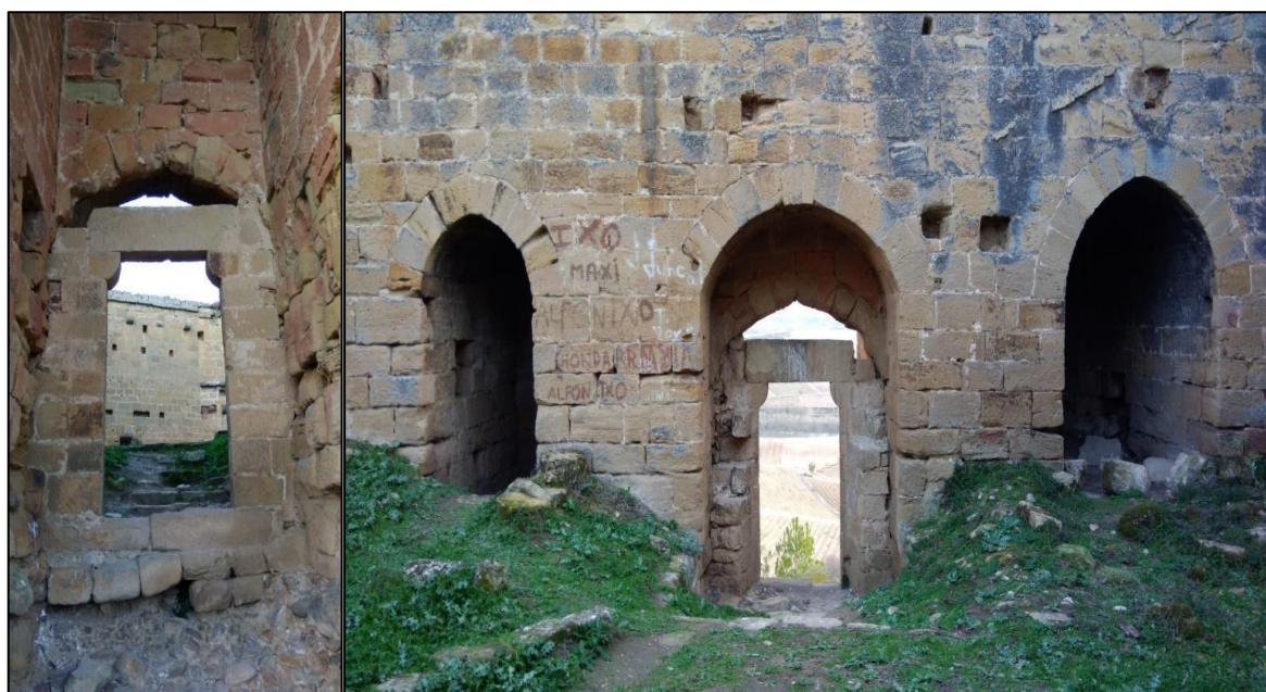
Figures 7-8. Main gate. Outside (left) and inside (right) (Photo credit: Authors).
