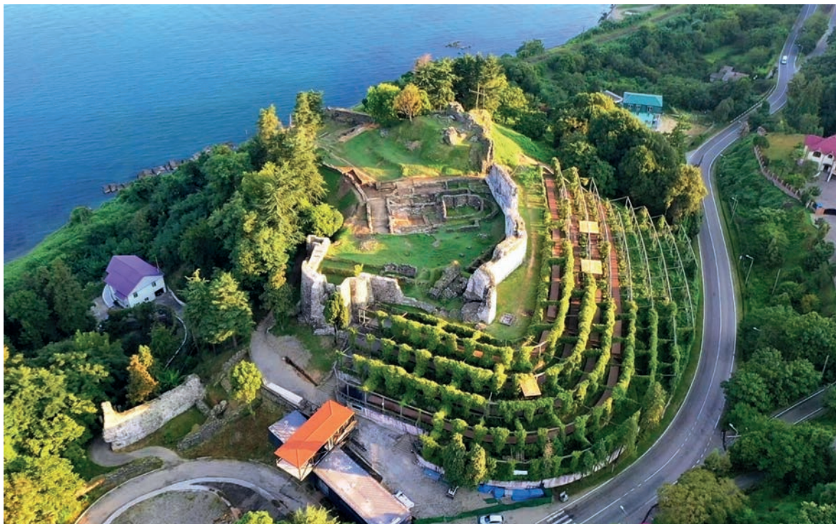
139. Petra from the air. Visible remains date from late antiquity and thereafter. The fort dominated the entrance into the Colchian plain proper. The town lies largely above the fort between the sea and the road into Colchis
