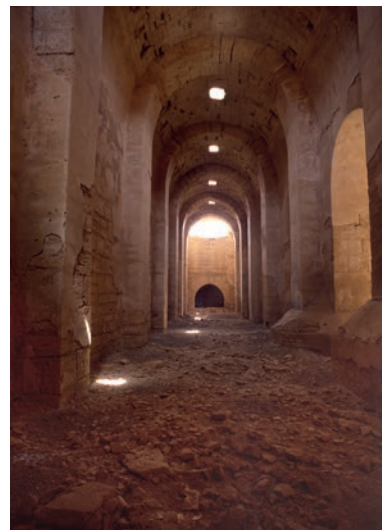
94. Resafa. Large vaulted cistern of the 6th century
