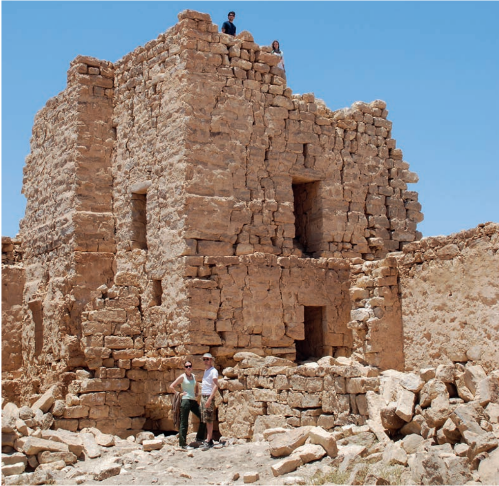
1. A corner tower at the fort of Qasr Bshir (Jordan)
