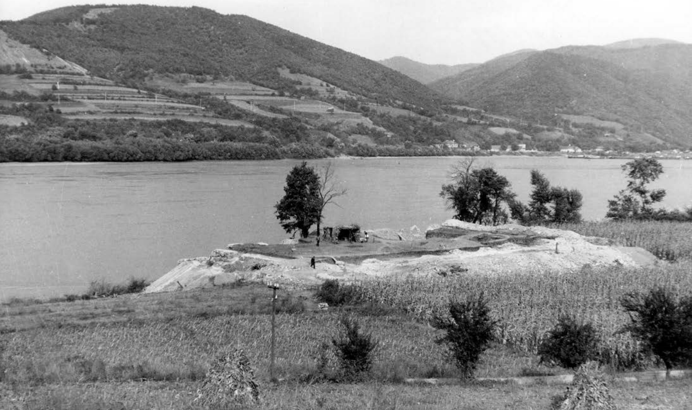
120. Fort Saldum during excavations 120. Utvrđenje Saldum tokom iskopavanja
