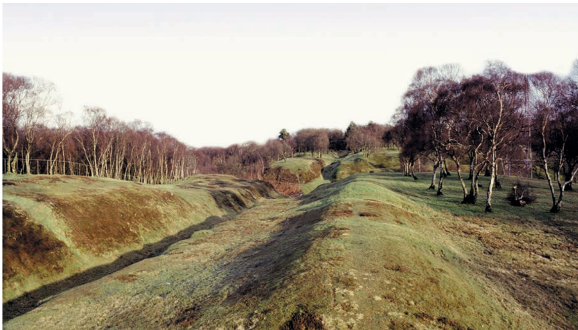
43. The Antonine Wall (Scotland, UK) was built of turf, which survives as a low mound; the ditch is to its left
