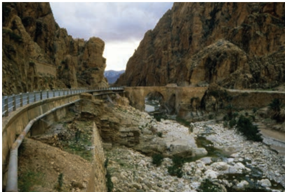
108. Roman bridge in the al-Kantara pass, connecting the Aures High Plains near Lambaesis with the pre-desert zone (Algeria)
