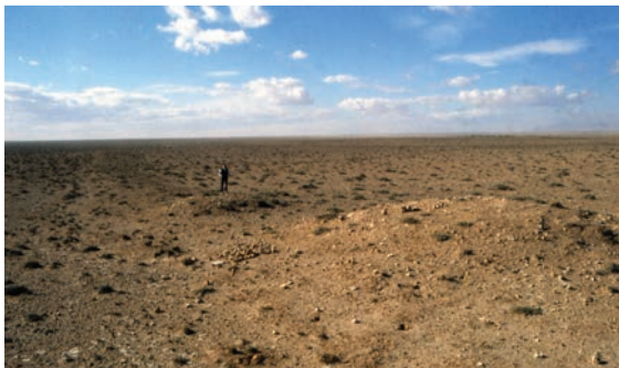
106. Double gate tower on the fossatum Africae near Gemellae (Algeria)
