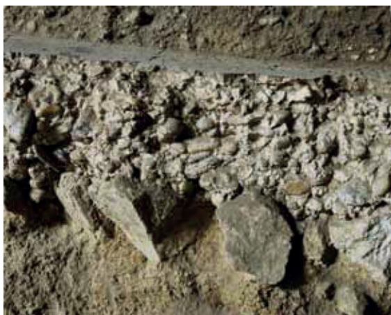
79. Vertical cut of the roman type pavement of the building 7/08
