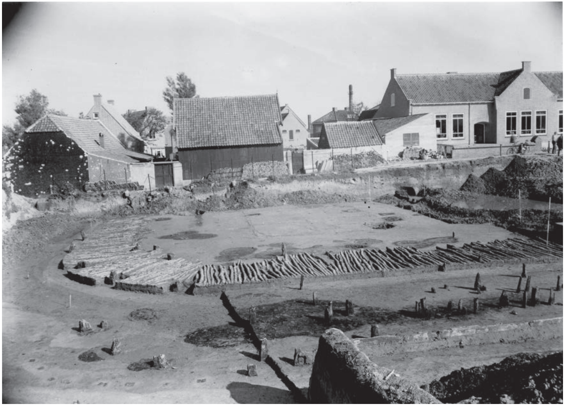
93. Excavation of Valkenburg in 1942 - Preservation of the ground beams.
