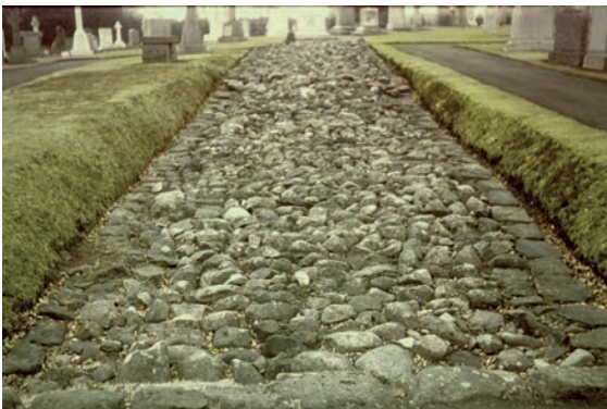
66. The stone base of the Antonine Wall in New Kilpatrick Cemetery, Bearsden. The base, 15 Roman feet (4.3 m) wide, is crossed by a drain
