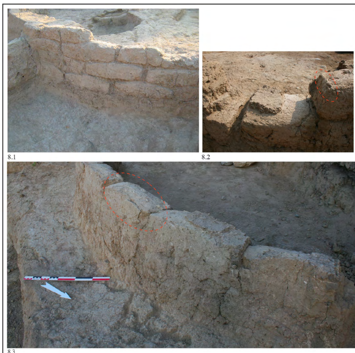
Figure 13. Molded plano-convex mud-bricks from Mentesh Tepe. a.: Detail of the four courses of mud-bricks, wall 293 (Sector 10) – View from the West; b.: Detail of the mortar between the mud-bricks, the wall 293 – View from the West; c.: Detail of the first course of mud-brick, wall 285 (Sector 15) – View from the North-East (after Baudouin et al. 2018: 58, fig. 8).
