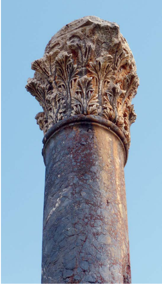
Figure 11: A column made of 'breccia' in the colonnaded street of Hierapolis Kastabala (Author)
