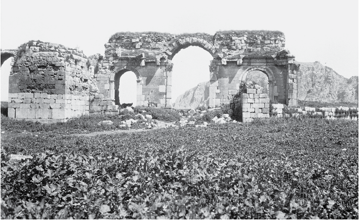
Figure 6: The Arch of Anazarbos before the collapse of the western passageway. Photograph by G.L. Bell, 20 April 1905 (© Gertrude L. Bell Archives, University of Newcastle-upon-Tyne, C_160)
