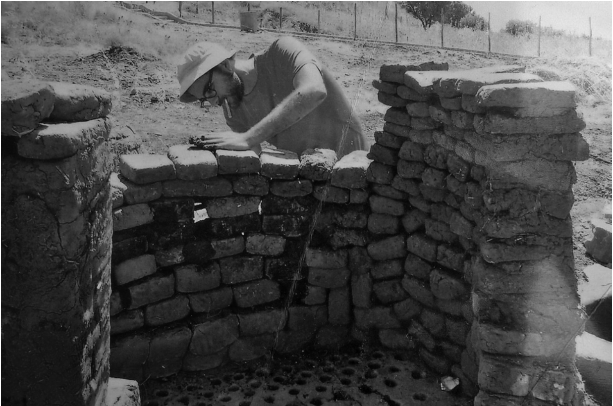
Figure 1: The author during the restoration of the kiln at the Parco Archeologico di Broglio di Trebisacce. Summer 2014 (photo by G. Pulitani)
