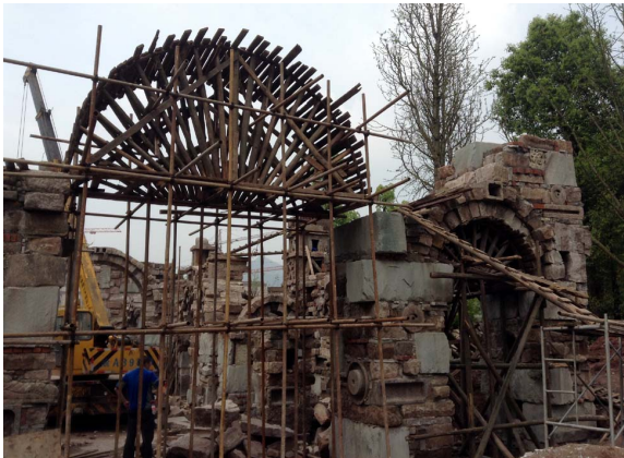
Figure 2-30 (bottom left), centrings for the construction site of a gate, Chongqing, China. Photograph by the author.
