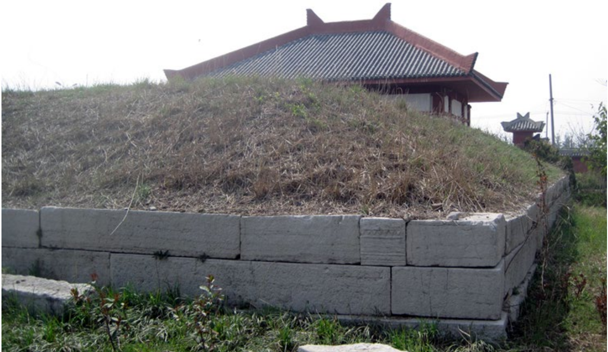
Figure 2-33, lined stone protection of the Baiji tomb. Photograph by the author.
