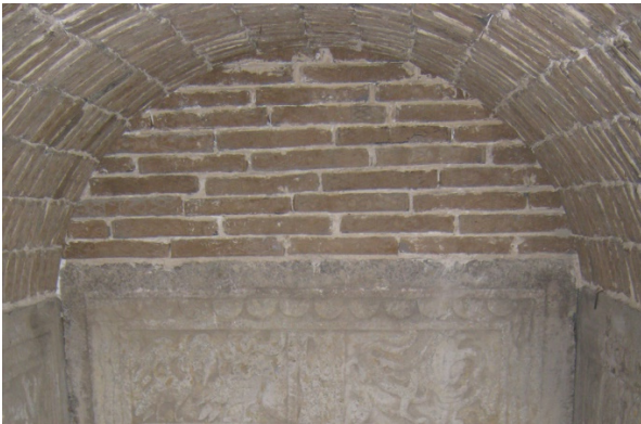
Figure 2-14a (top left), round dome vault of the Jianhe tomb near Luoyang.
