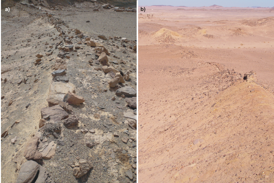
Fig. 30 a) Presumed canal on top of Wall C with two faces on each side (view towards the south). b) Wall D. There is no indication of any canal-like structure on top of this wall, which could provide transportation of water from the rock into the settlement (view towards the north).
