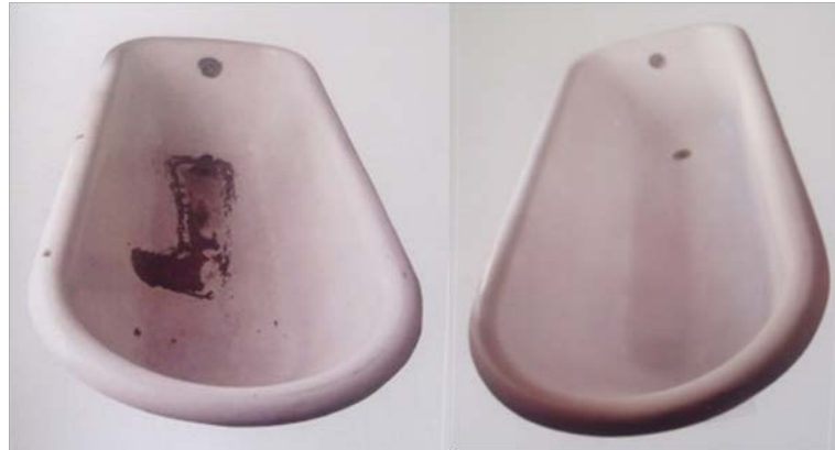
Fig. 18. Before and After Restoration
