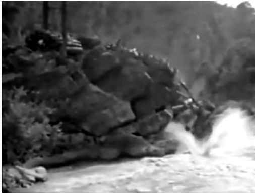
Fig. 4 Rolling a Stack of Logs into River (Okay Sütçüoğlu Archive)
