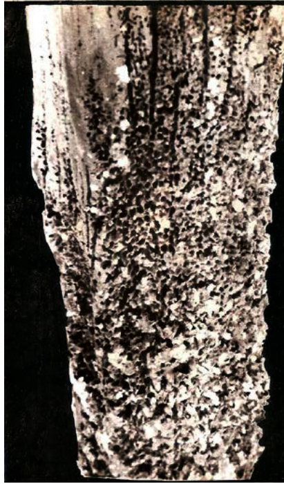
FIGURE 16: A JETTY PILE OF 'MATTI'(TERMINALIA SP.) HEAVILY DAMAGED BY PILL-BUGS AND PIDDOCKS AT THE INTERTIDAL AREA (LOCALITY : KARWAR, INDIA).
