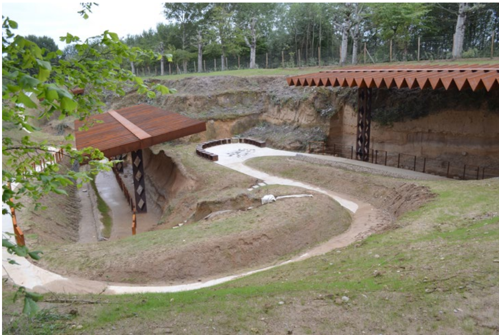
FIGURE 3. THE MAIN GEOLOGICAL PROFILE AT VELDWEZELT-HEZERWATER, WHICH INCORPORATES THE REMAINDERS OF ALL THE MAJOR ARCHAEOLOGICAL HORIZONS, IS NOW PROTECTED BY THE CHARACTERISTIC ROOF CONSTRUCTIONS.
