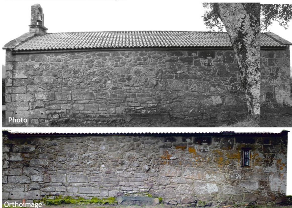
FIGURE 4. DIFFERENCES IN THE SOUTHERN ELEVATION OF THE CHAPEL OF SAN MAMEDE DOS MÁRTORES: TOP, A PHOTO OF THE ELEVATION WITH A TREE THAT HIDE S PART OF THE SURFACE, AS WELL AS SUFFERING FROM THE TYPICAL DEFORMATION SEEN IN PHOTOS; BOTTOM, THE ORTHOIMAGE OF THE SAME ELEVATION, WITHOUT ANY DEFORMATION OR THE TREE IN FRONT OF THE FAÇADE.
