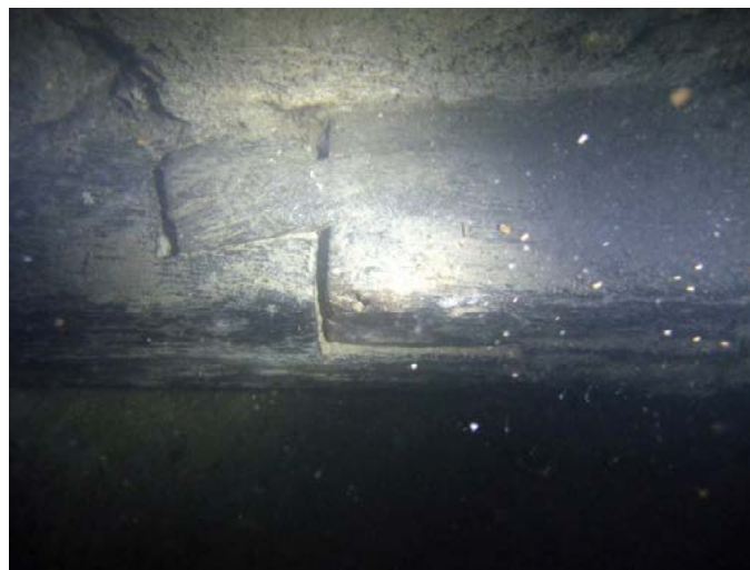
FIG. 24. WOODEN BEAMS IN THE BASE OF THE SOUTH-EASTERN WALL OF TOWER 1
