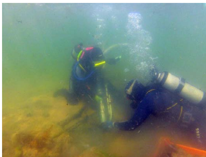
FIG. 20. DIGGING OF TOWER 1 WITH THE AIRLIFT
