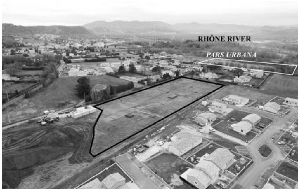
FIG. 2. AERIAL VIEW OF THE SITE (GENTIL-PERRET J. P., INRAP).
