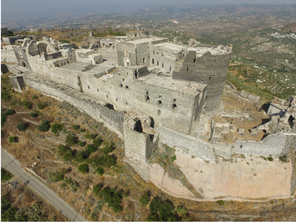
Figure 1.5. Margat: citadel from the south-west, with the outer wall and the gate tower Ti of the early Hospitaller period in the foreground and behind it the western façade of the citadel with the following buildings from left to right: inner gate tower (F), J, M, chapter house (Ch), kitchen (D), N. Behind it the buildings of the church (H), K and the donjon (L) can be seen from left to right (photo: B. Takáts).
