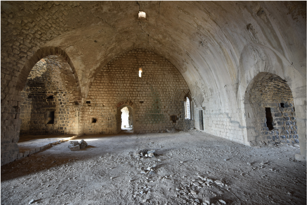
Figure 1.9. Margat: first-floor room (L2) of the donjon looking north with the sleeping alcove in the left, putlog holes and consoles of the wooden mezzanine floor and numerous cupboard niches in the walls.
